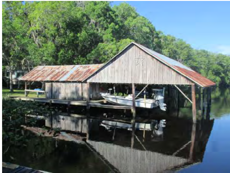
Photograph 1 East Facade of Boathouse
