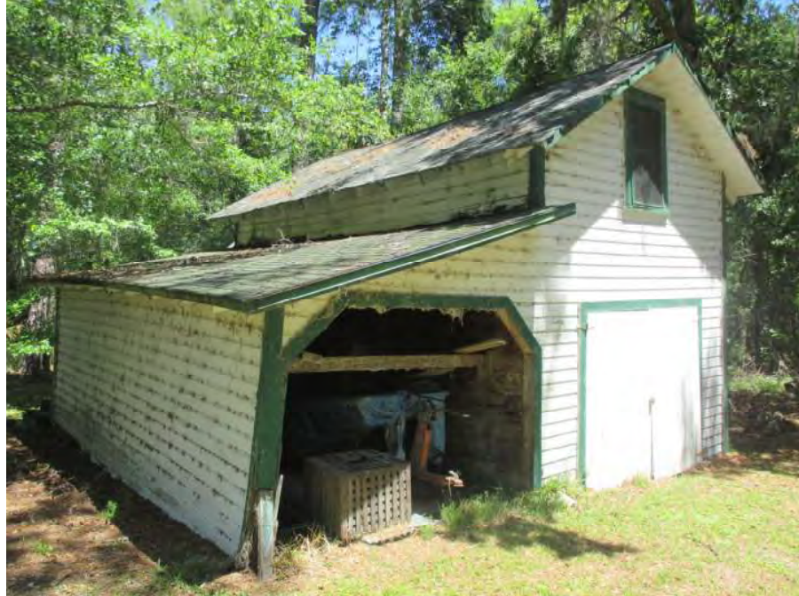
Photograph 1 Overall Attic Garage
