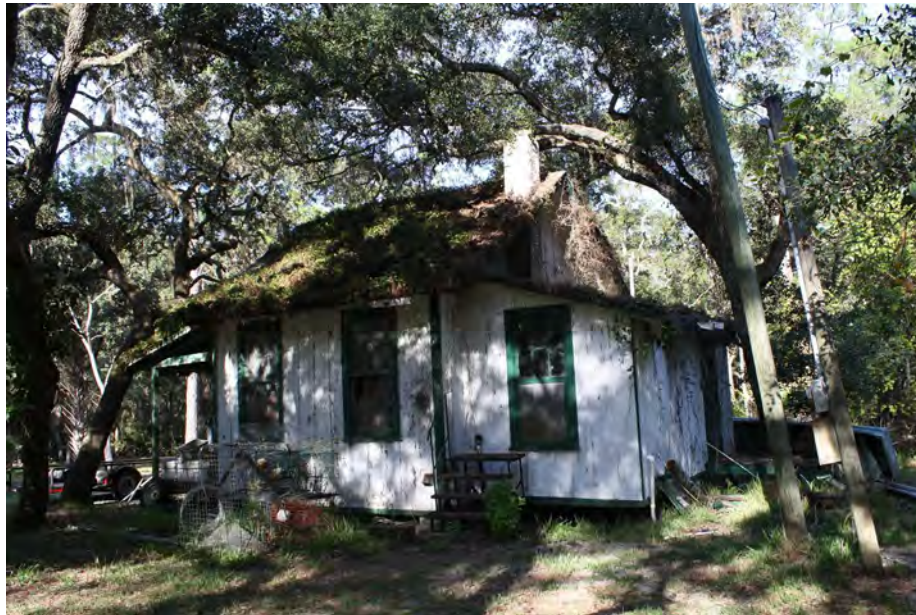
Southwest corner of the Cook's House
