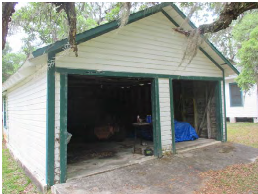
Photograph 1 Overall Double Garage Entry
