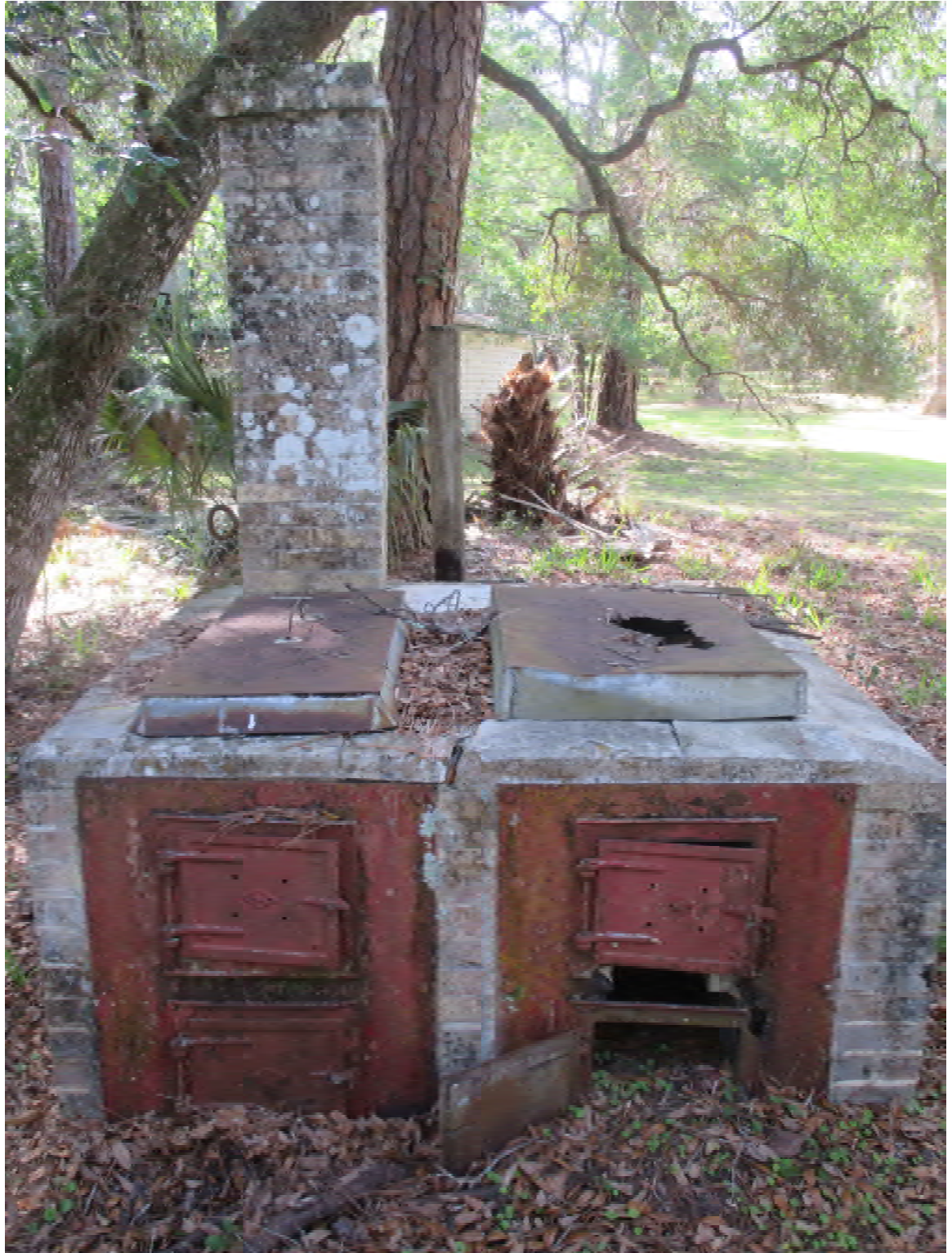
Photograph 1 Overall Outdoor Grill Front
