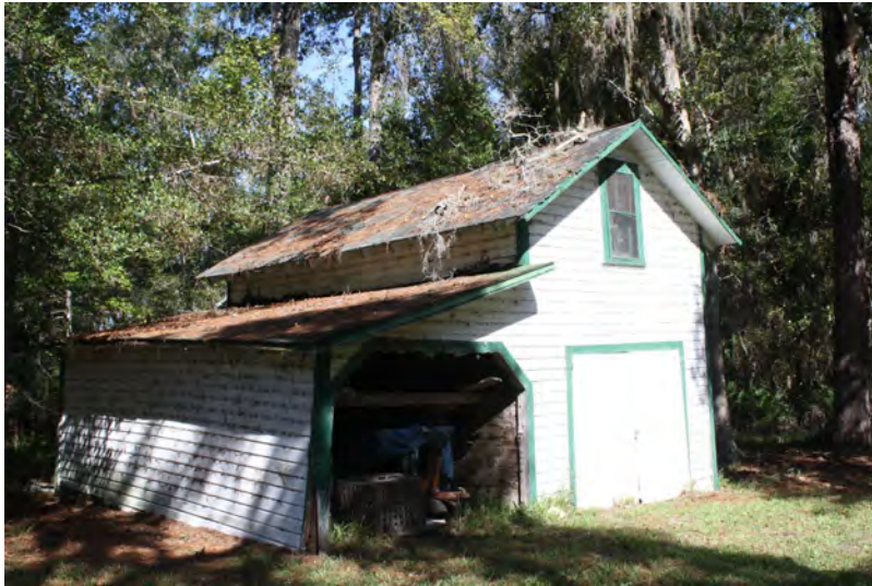
Front of Attic Garage.
