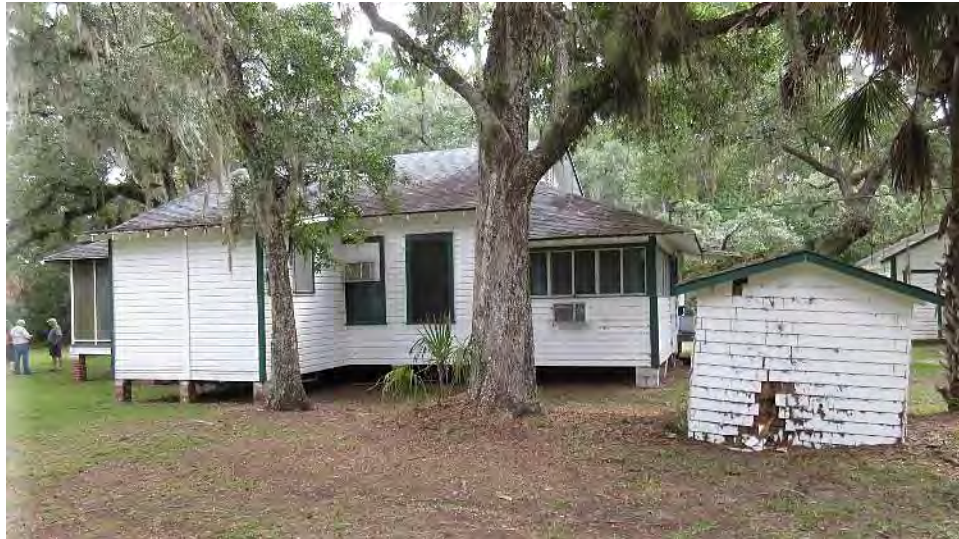
View of the west façade.
