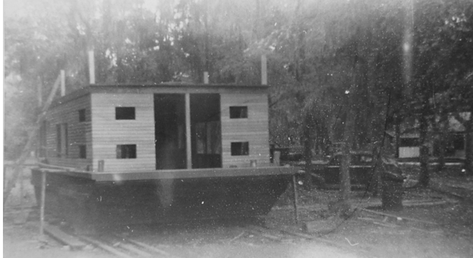
Circa 1939 or early 1940 view of the Houseboat deck under construction. (Photo courtesy Bob McKinstry)
