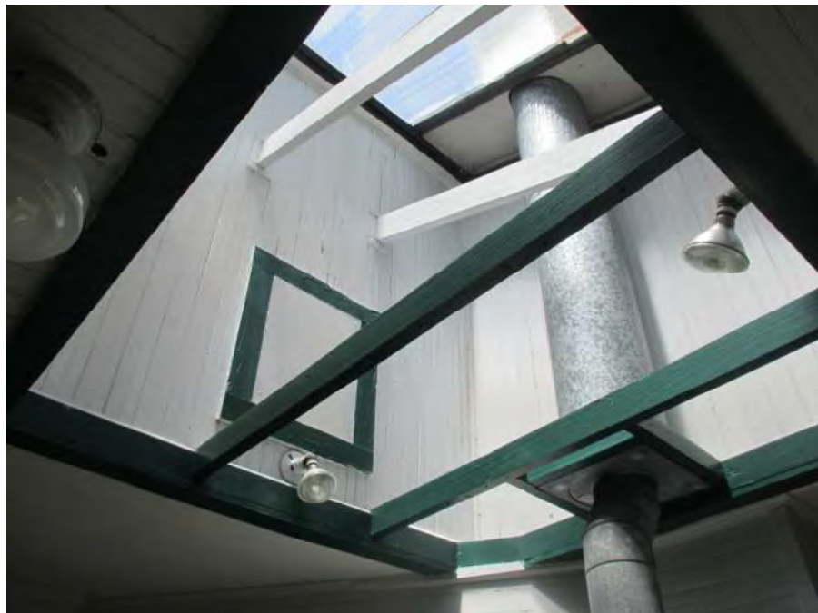
Photograph 3 Skylight within Main House Kitchen
