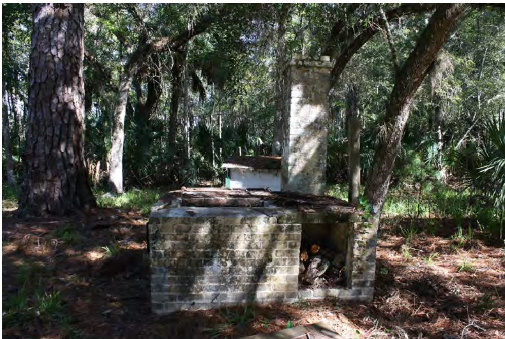
West side elevation of the grill.
