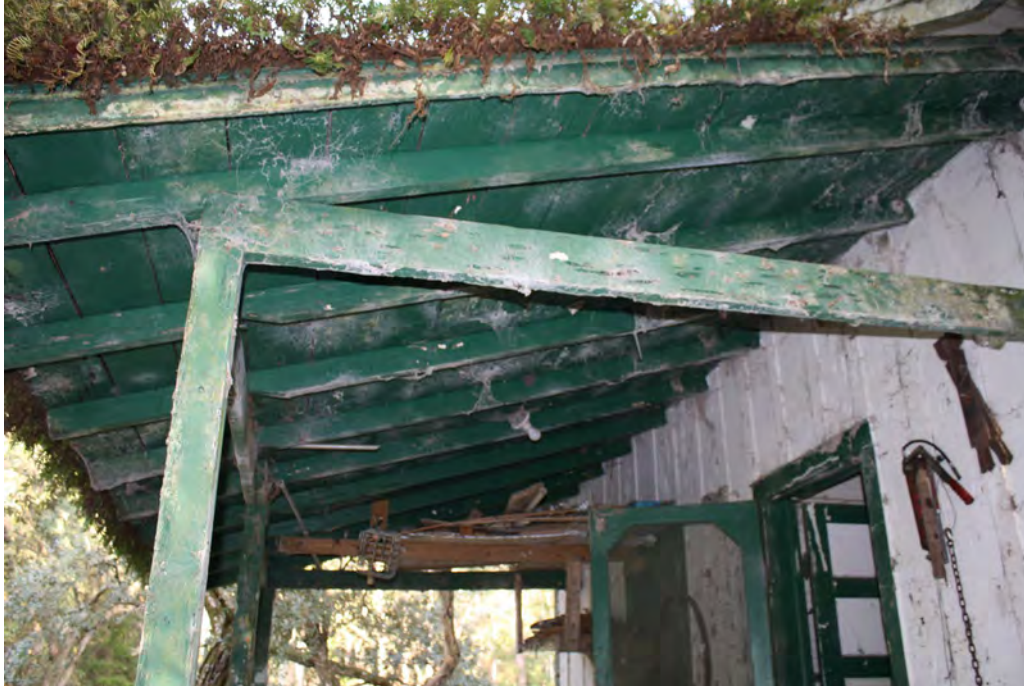
Porch framing detail.
