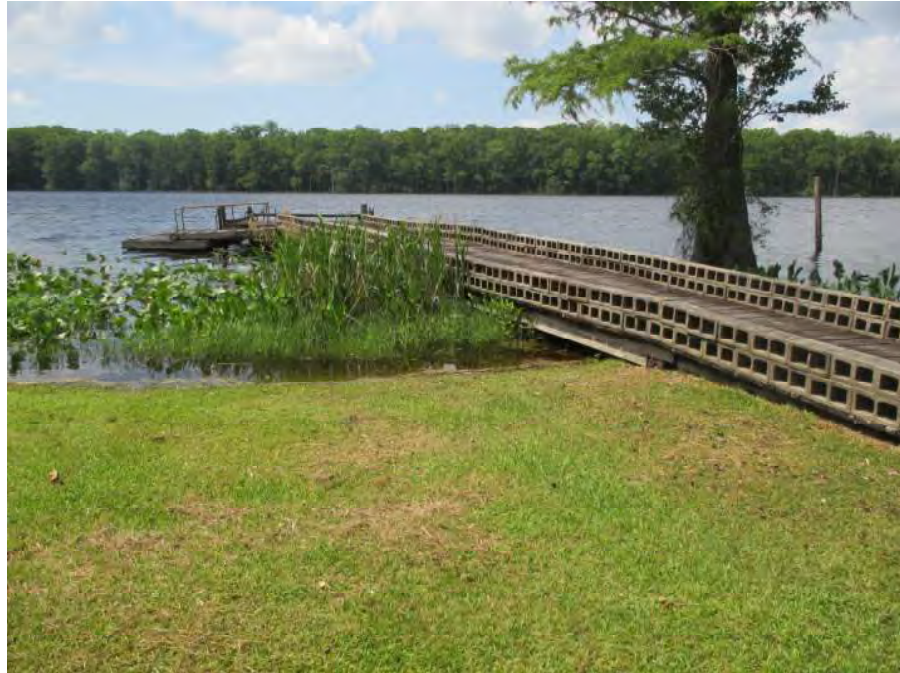
Photograph 1 Overall of Dock
