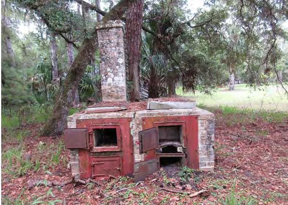
View of the Cahill fireboxes at the front of the Grill.
