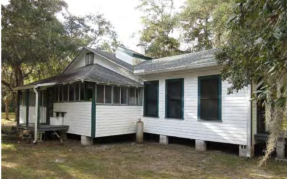
View northeast of the rear of the building. Note the skylight and chimney.
