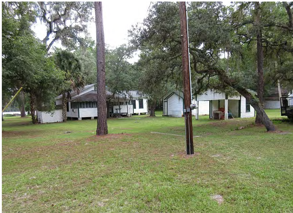
View of the central portion of the Vista compound toward the rear of the Main House.
