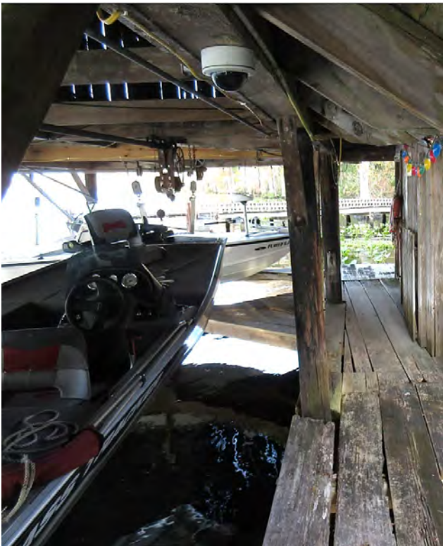
Vista Physical Description
