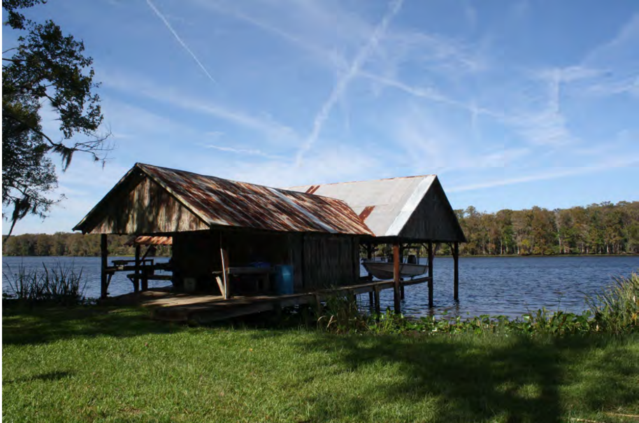
The Boathouse from the south side showing fish area and shed.
