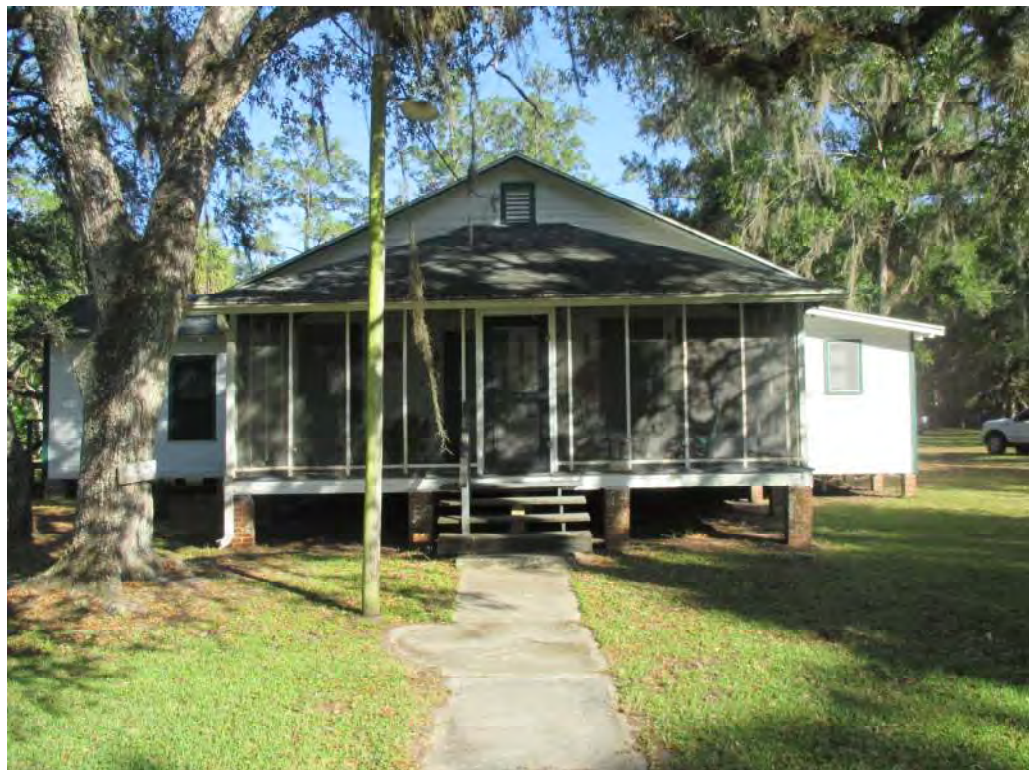
Photograph 1 Primary Facade of Main House
