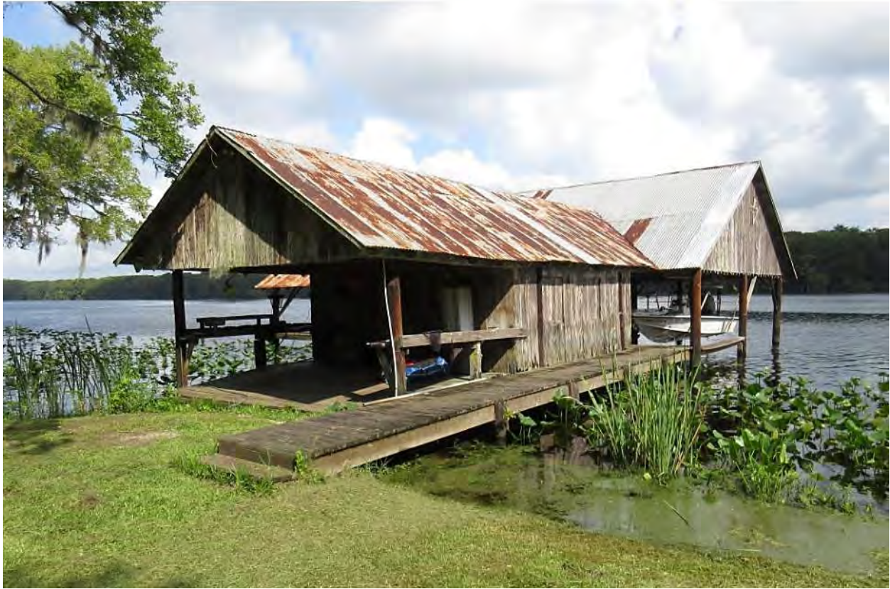
The primary (south) and east facades of the Boathouse.
