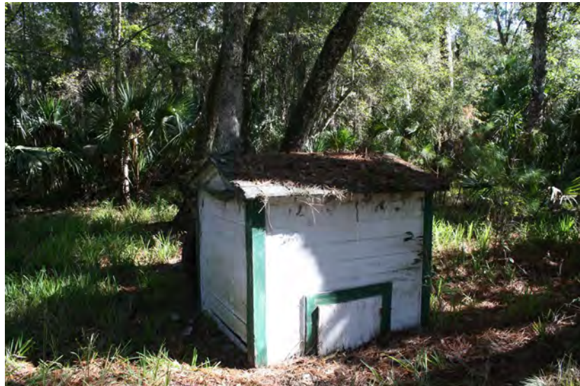
The smoker needs some repairs, most notably at the ground level.
