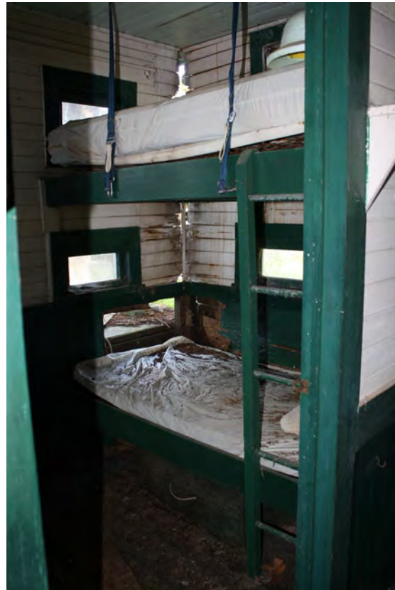
Berth area on right side. This is one of the worst areas of the boat and will be restored.
