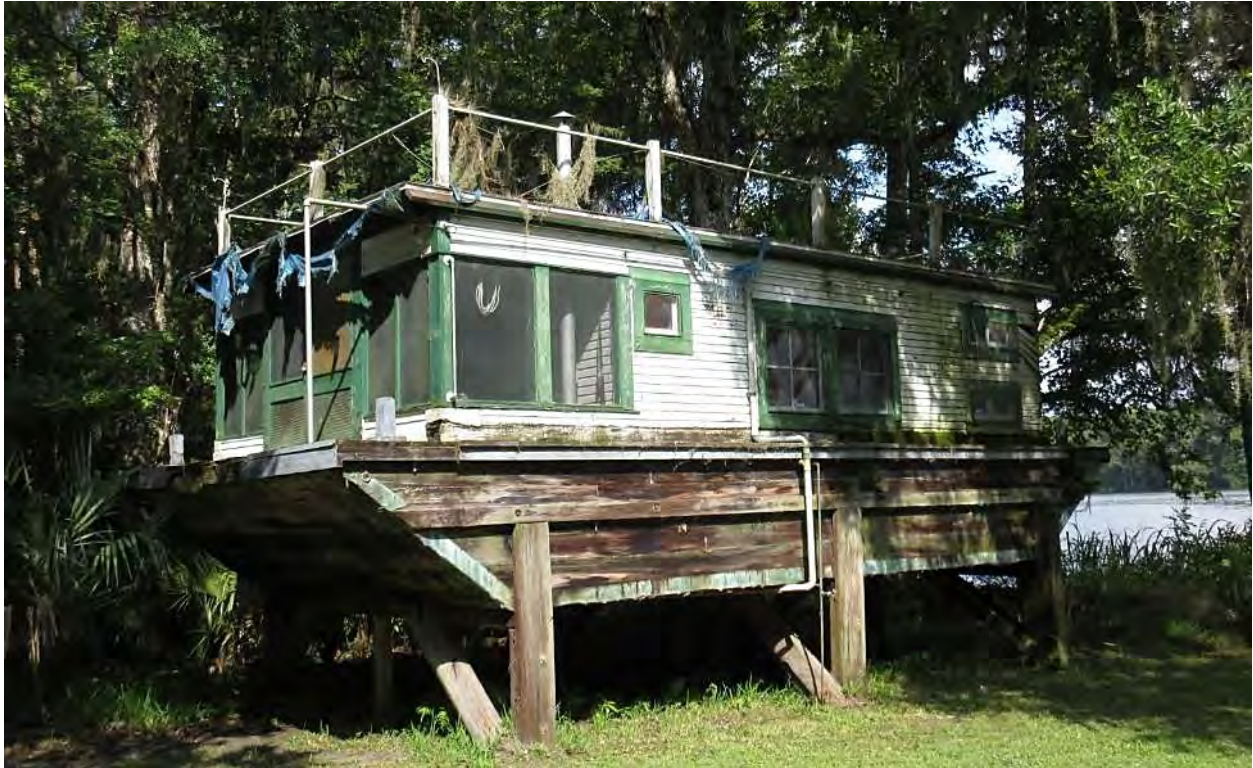
View northwest of the Houseboat.
