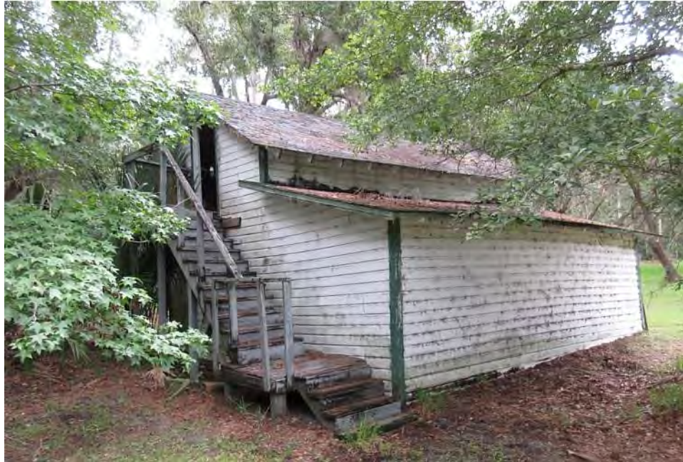
The rear (north) and west facades.
