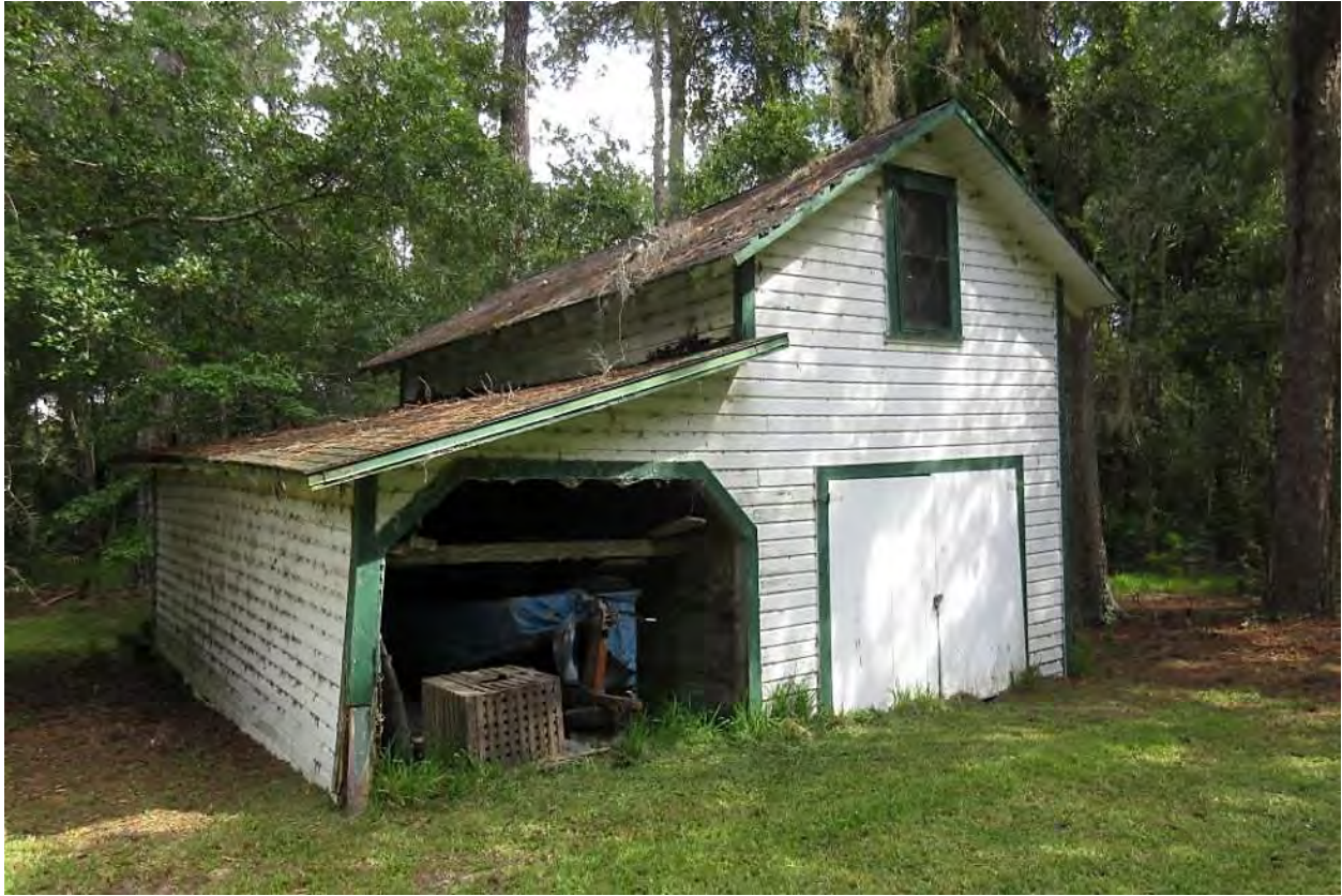
View northeast of the Attic Garage.
