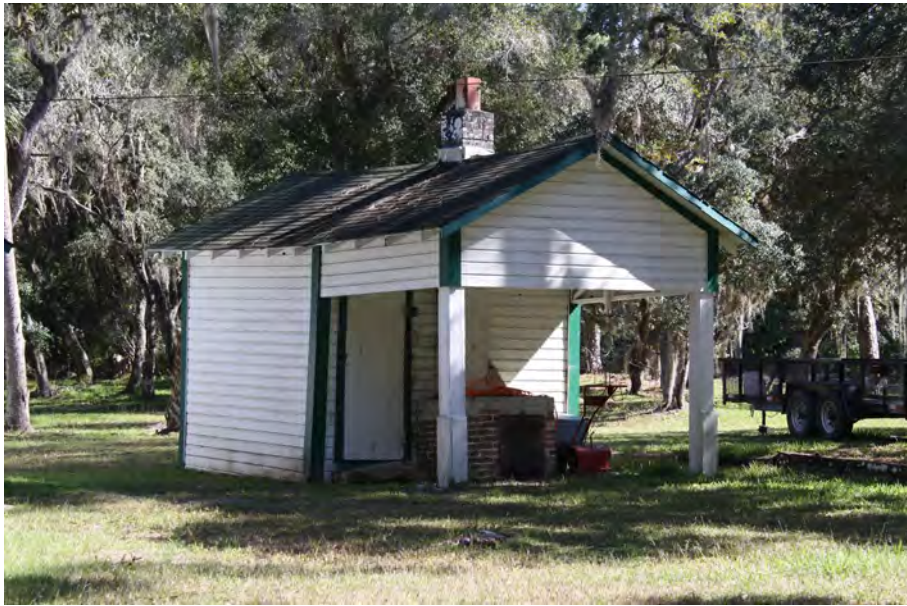
Fryer Shed from the west side.
