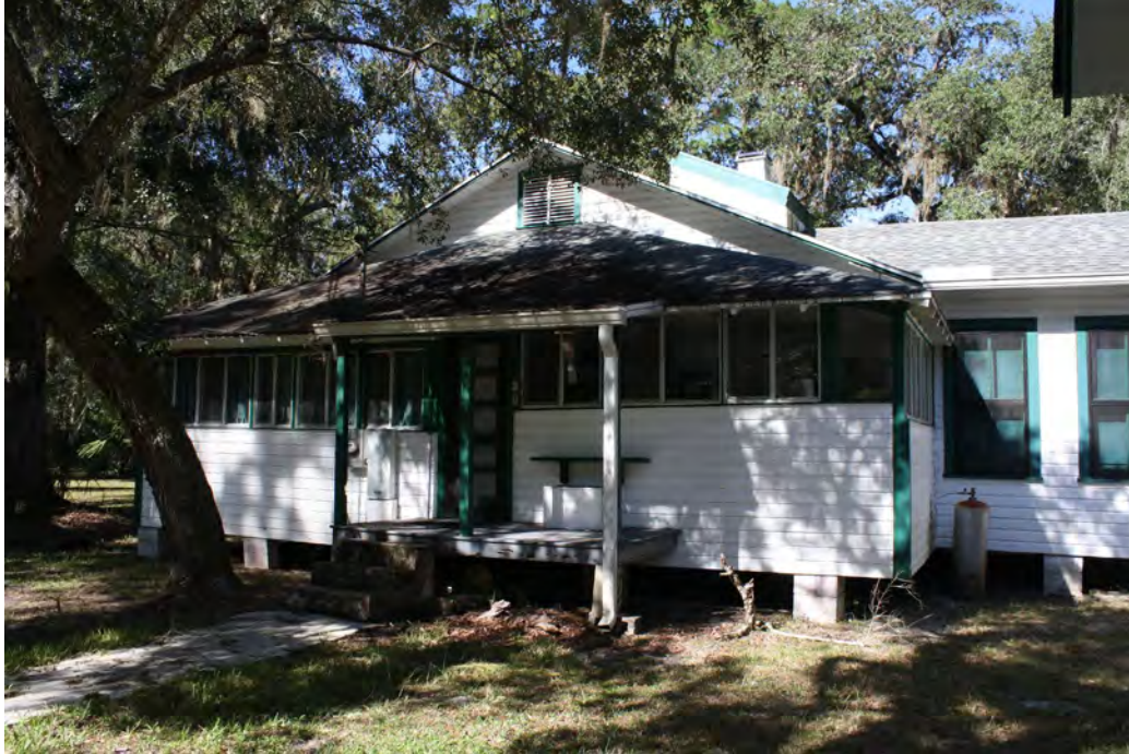
South elevation of the Main House. This elevation shows later additions, including the south porch, it's enclosure with glass windows, extension to the east, and dining room addition.
