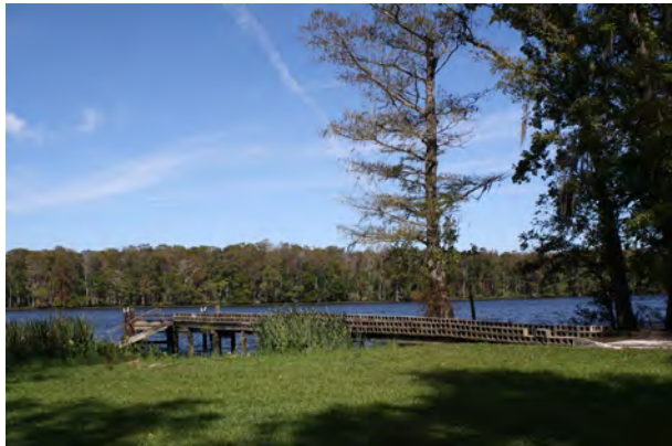
Pier leading to the Docks.
