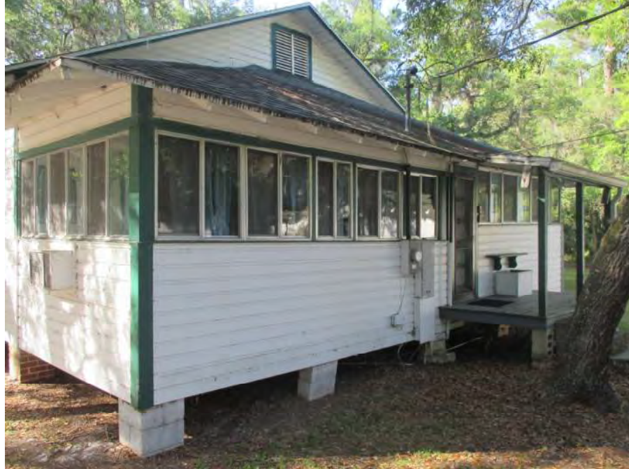
Photograph 2 Southwest Corner of Main House
