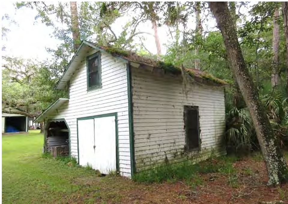
The primary (south) and east facades.
