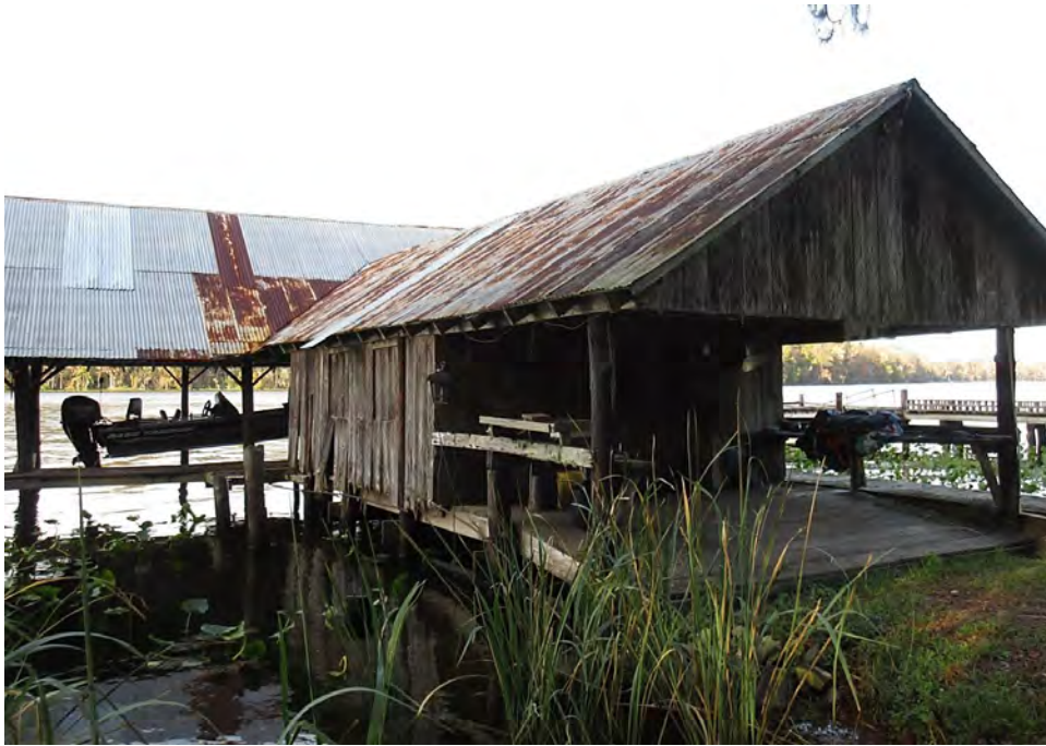
Partial view of the west façade of the Boathouse.
