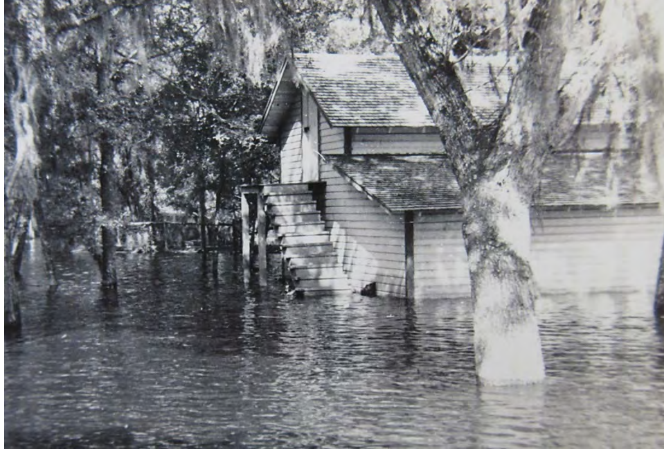
View of the east and rear facades of the Attic Garage during the April 1948 flood. (Photo courtesy Bob McKinstry)
