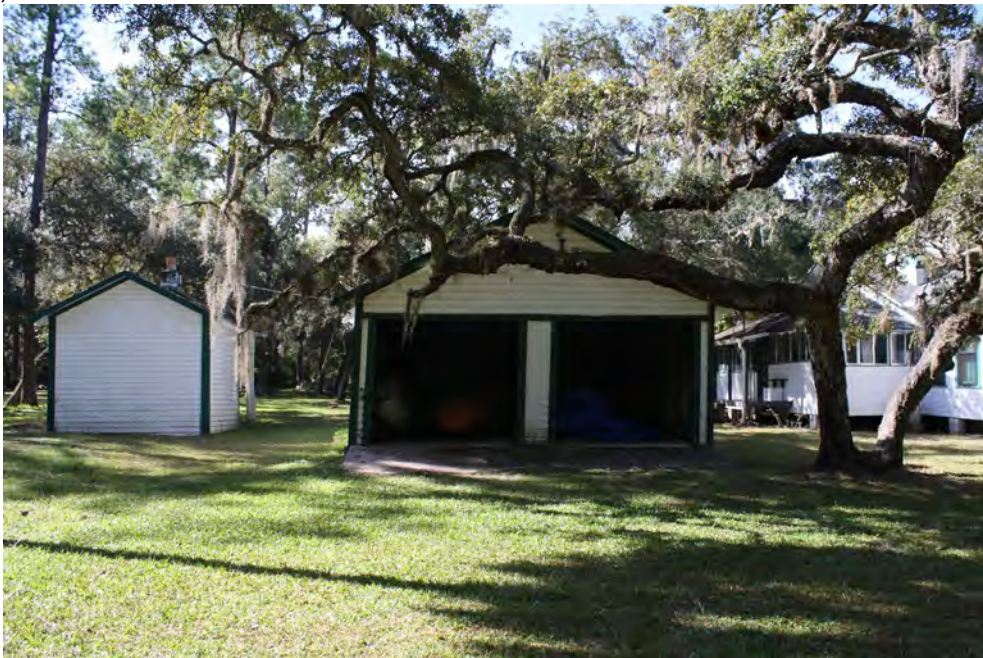
The double garage entrance.
