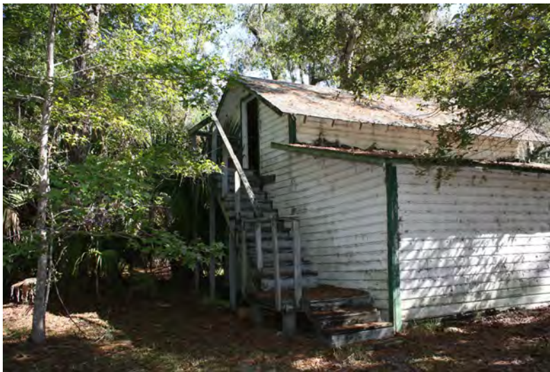
Rear of Attic Garage.
