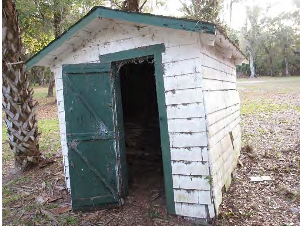
Detail view showing door construction.
