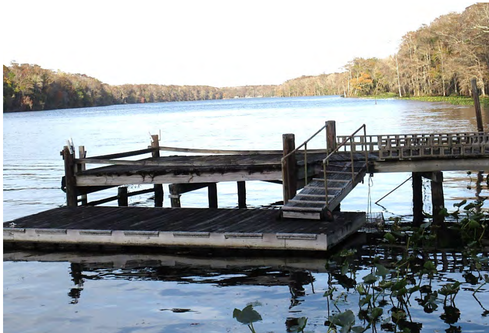
View east upriver from the Boathouse to the Dock.
