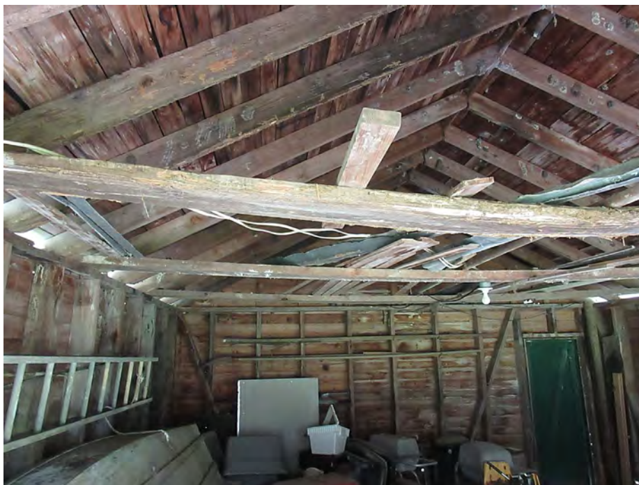
Detail of the garage walls and ceiling.
