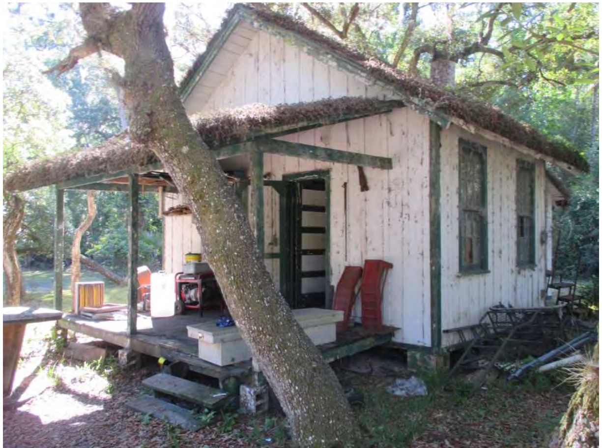
Photograph 1 Cook's House Main Entry Porch
