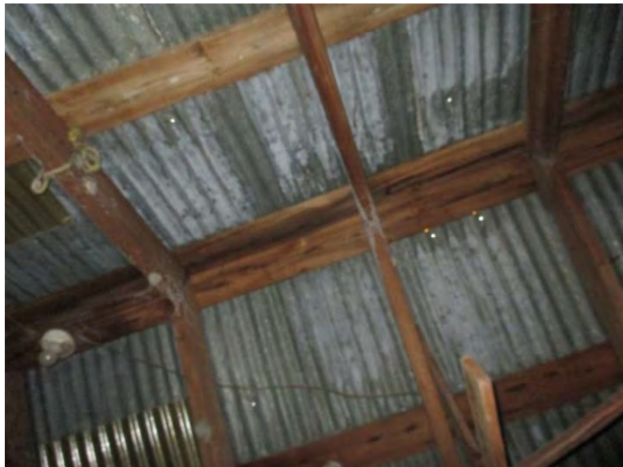
Photograph 4 Underside of Metal Roofing
