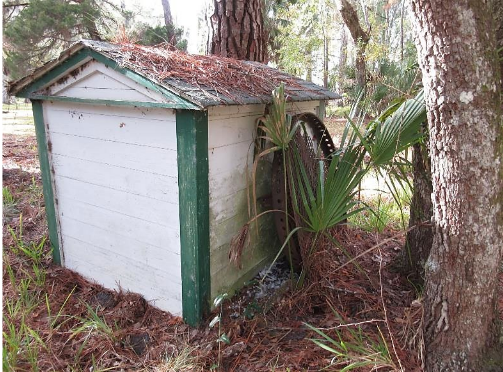
View toward the south and east sides of the smoker.
