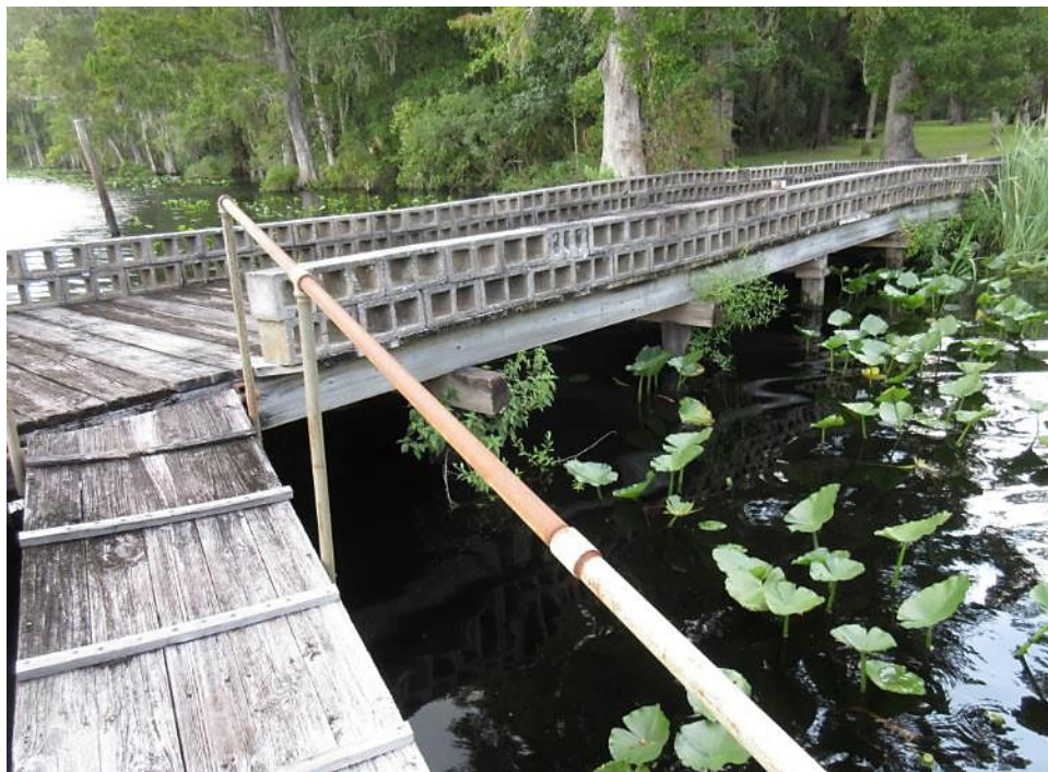
View east from the floating dock toward the fixed finger of the Dock.
