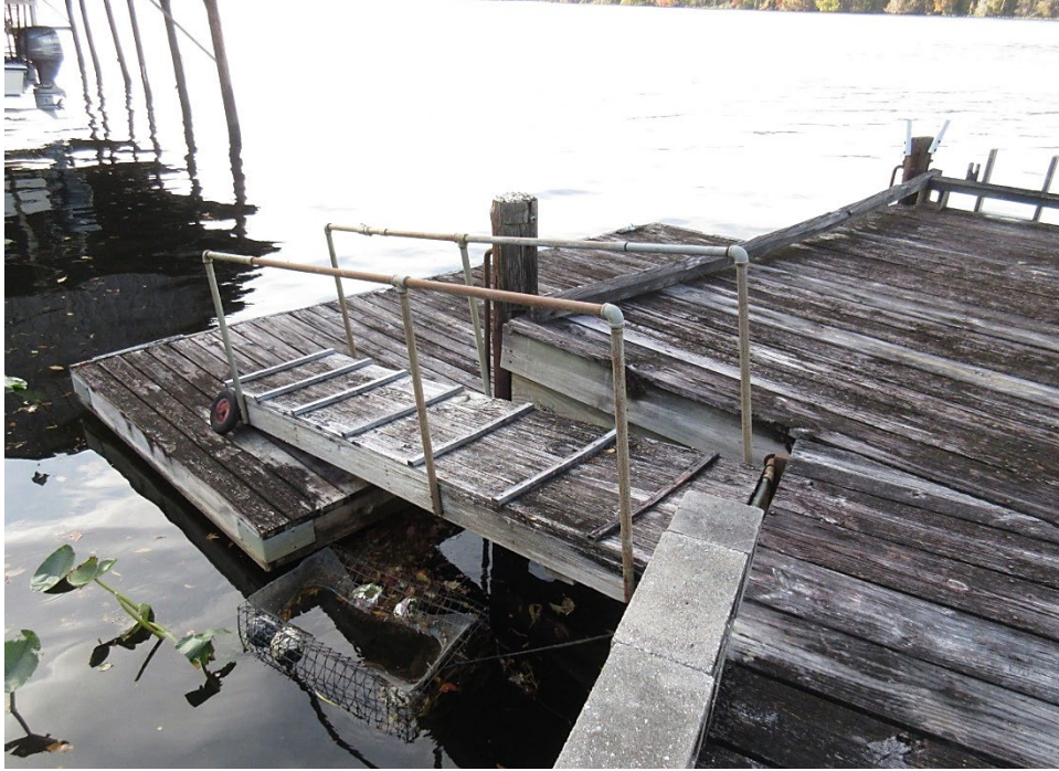
View northwest toward the ramp down to the floating portion of the Dock.
