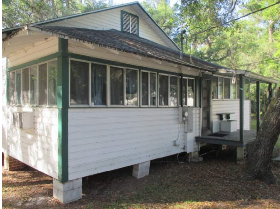
Photograph 2 Southwest Corner of Main House
