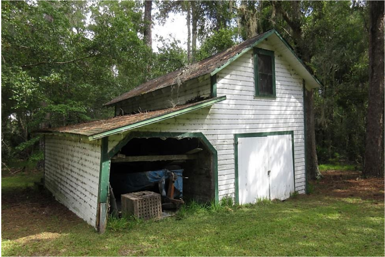
View northeast of the Attic Garage.
