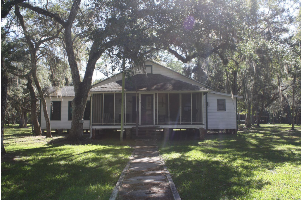
North elevation of the Main House in November 2019
