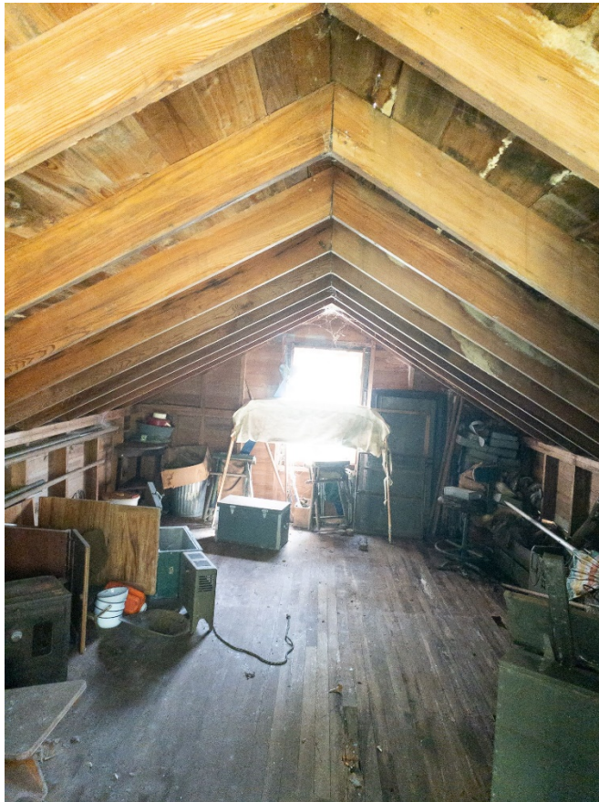
Attic of Attic Garage.
