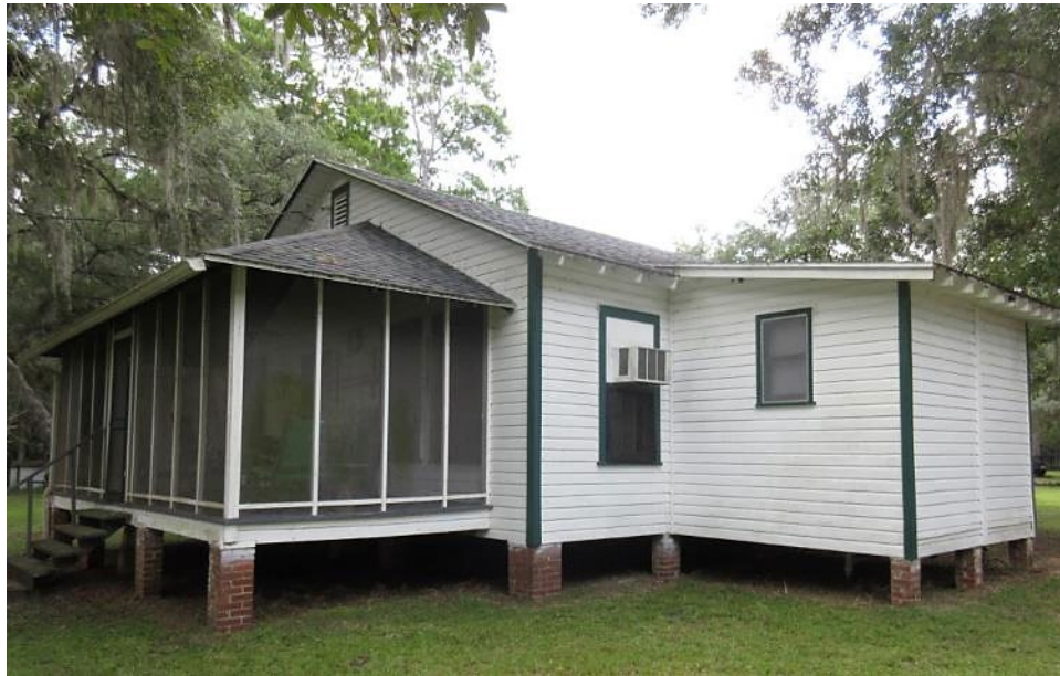
View of the northwest corner of the Main House.
