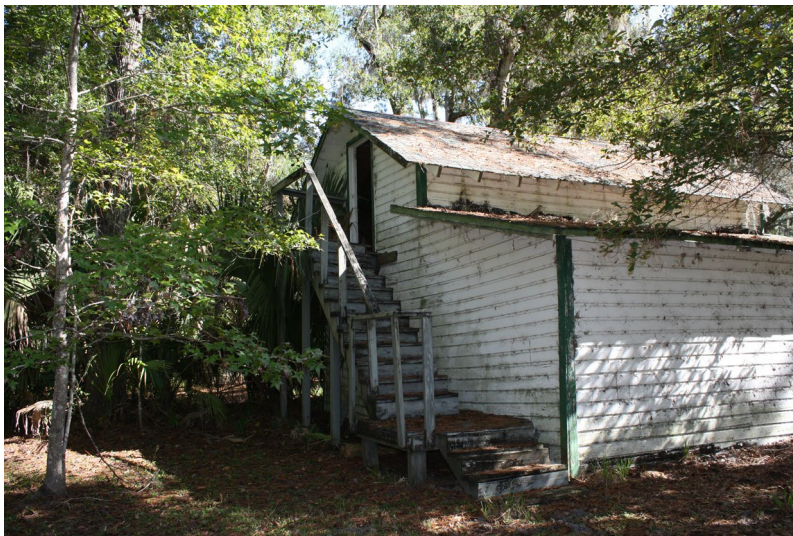
Rear of Attic Garage.
