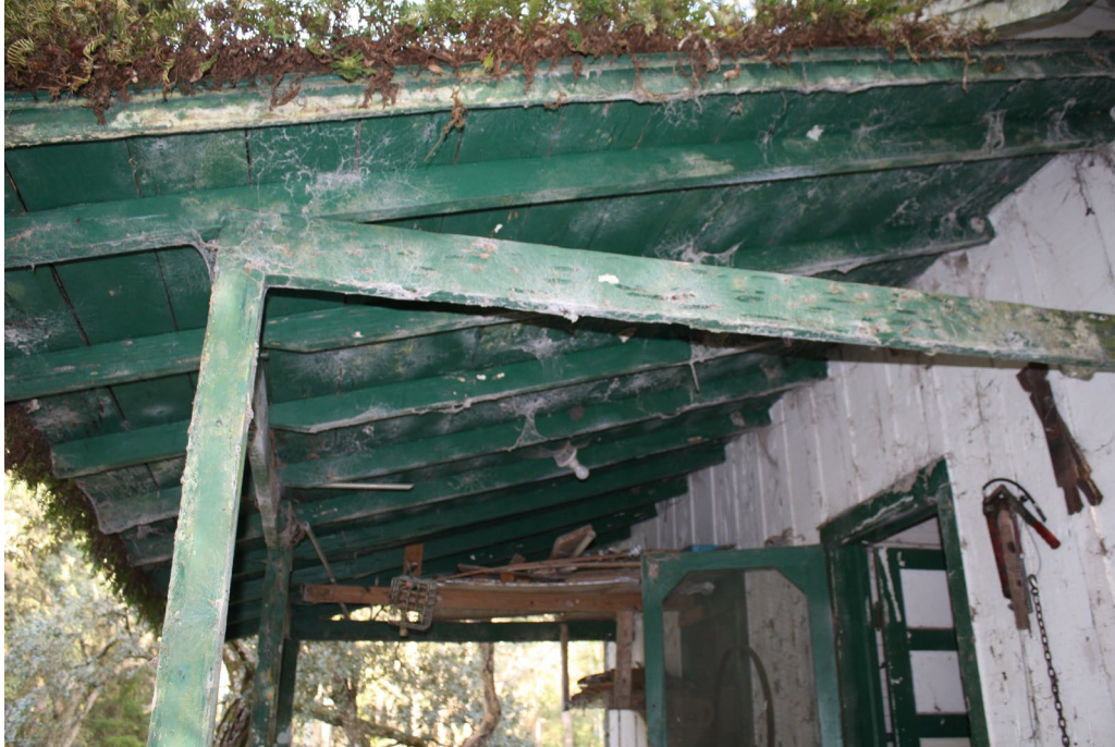
Porch framing detail.
