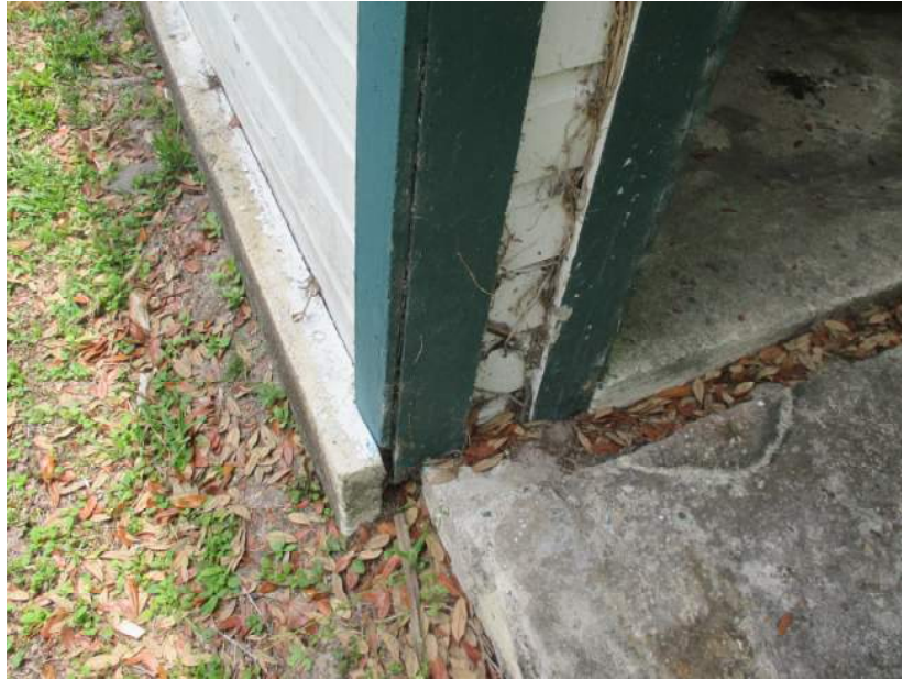
Photograph 8 Hinged Concrete Entry Ramp to Interior Slab
