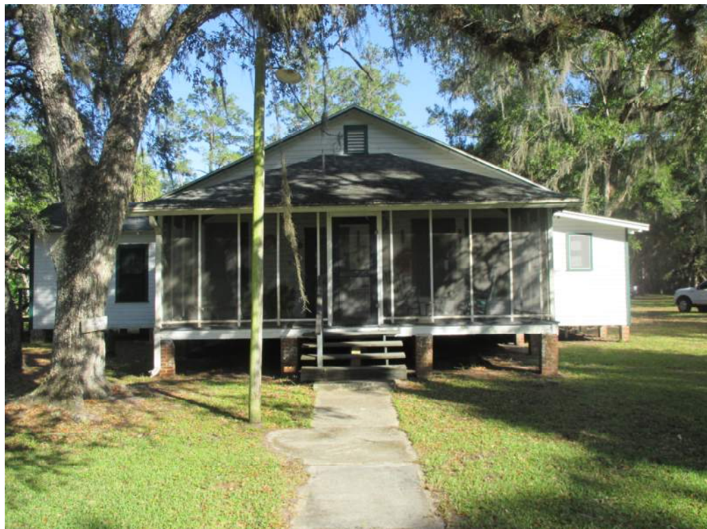
Photograph 1 Primary Facade of Main House
