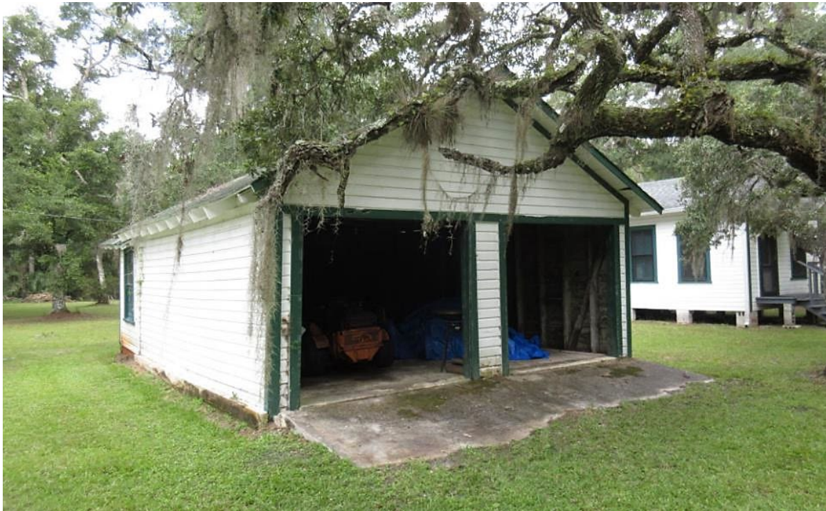
Primary (east) and south facades of the Garage.
