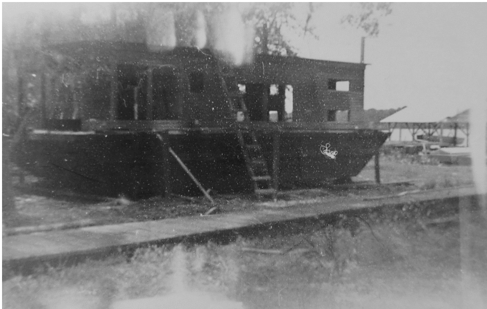
Circa 1939 or early 1940 view of the Houseboat deck under construction. Note the first portion of the Boathouse has been completed. (Photo courtesy Bob McKinstry)
