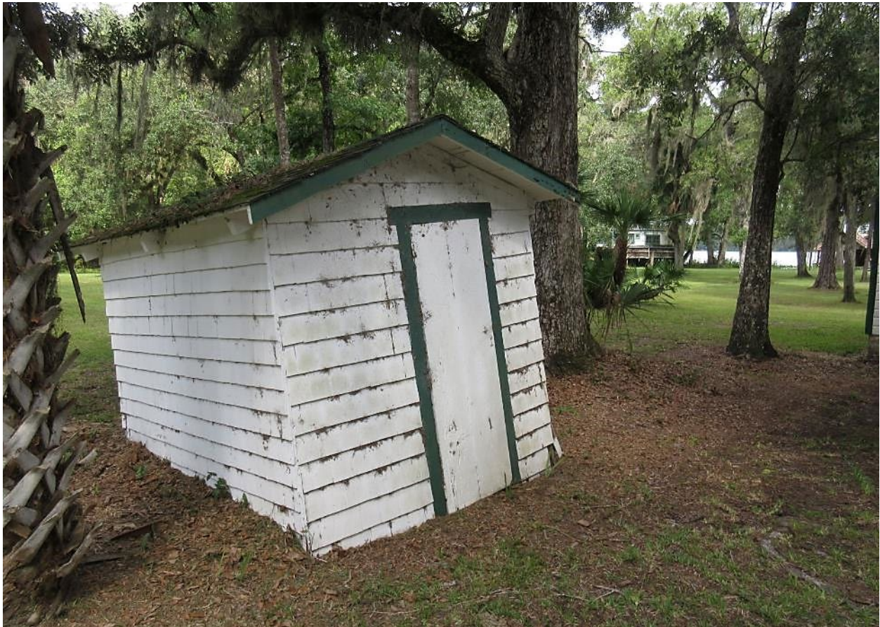
South and east sides of the Woodshed.
