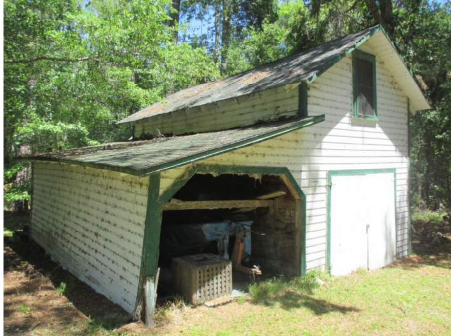
Photograph 1 Overall Attic Garage
