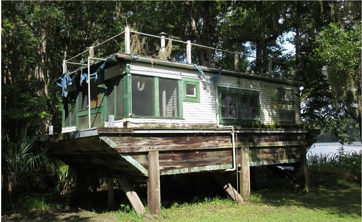
View northwest of the Houseboat.
