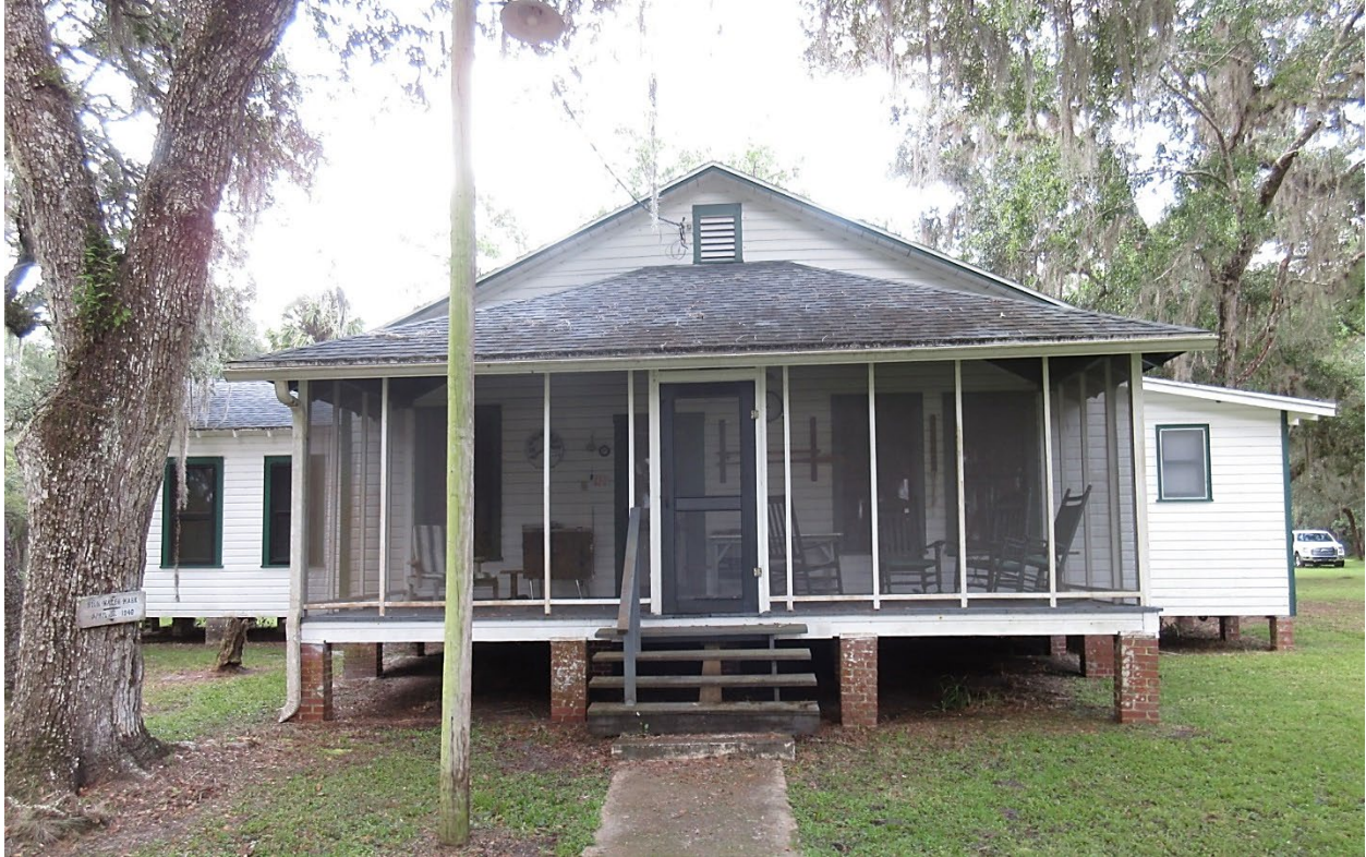
View south of the primary façade of the Main House
