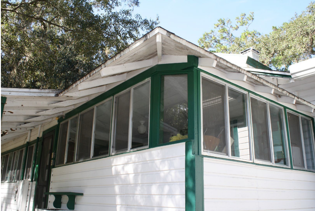
Detail of the south porch addition showing the east side extension.
