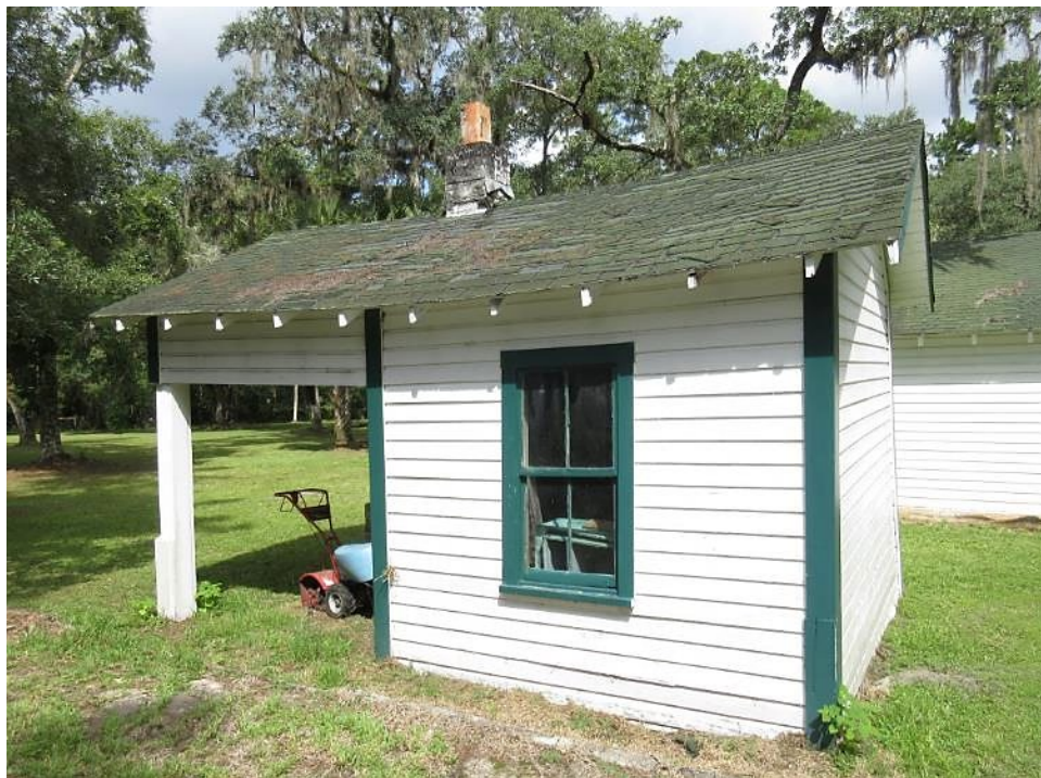
View north of the south façade of the Fryer Shed.
