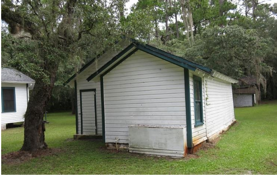
Rear (west) and south facades of the Garage.
