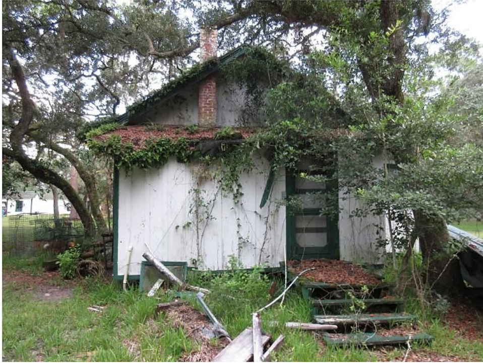
Rear (south) façade of the Cook's House.
