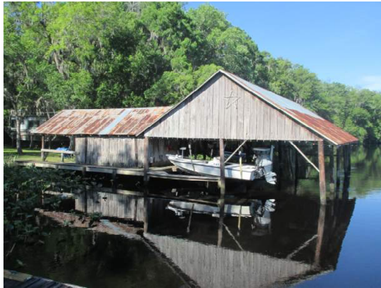
Photograph 1 East Facade of Boathouse
