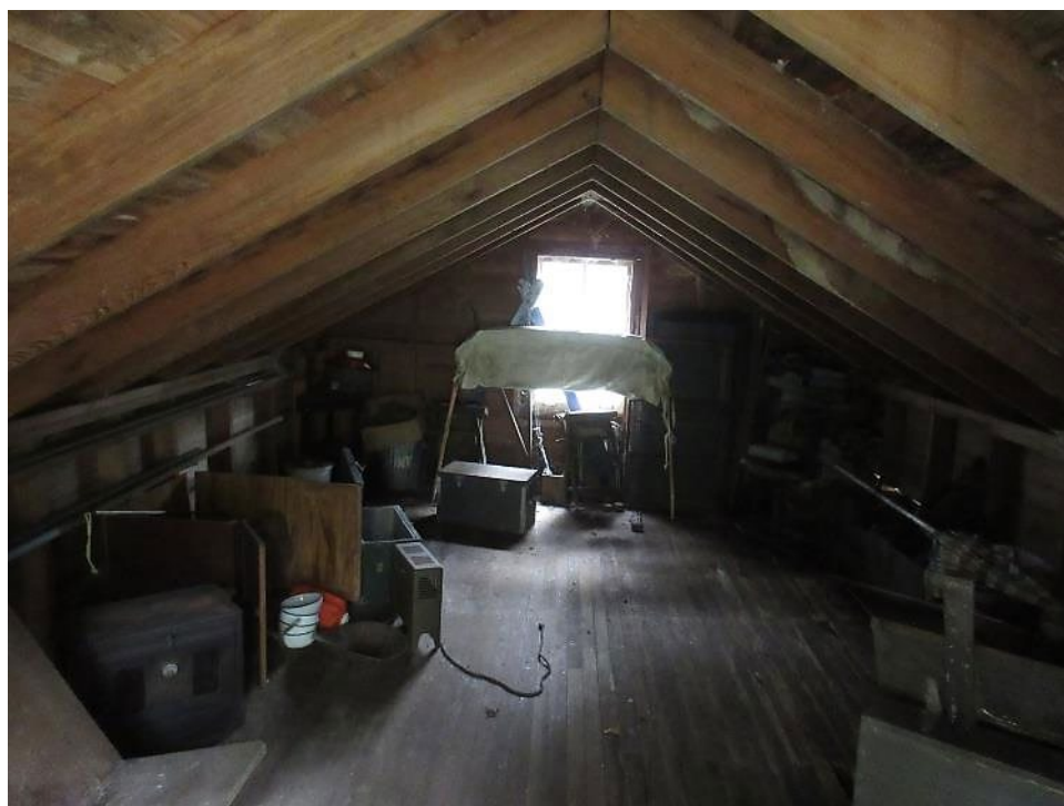
Interior of the Loft garage.
