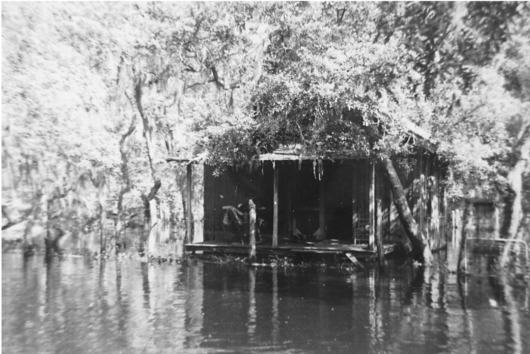
View of the Cook's House during the April 1948 flood. Note that the trees presently framing the building are already mature by that time. (Photo courtesy Bob McKinstry)
