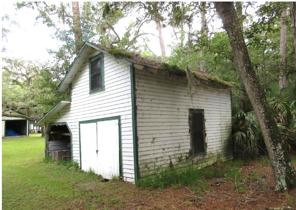
The primary (south) and east facades.
