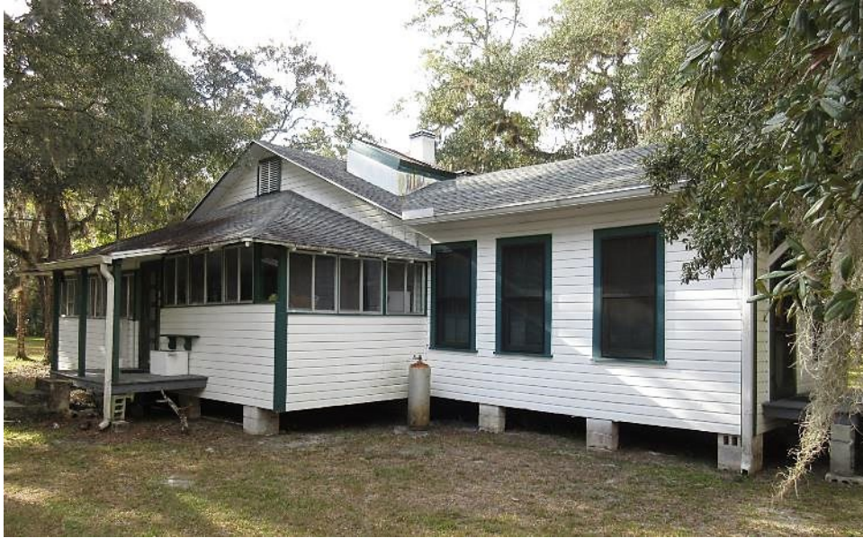
View northeast of the rear of the building. Note the skylight and chimney.
