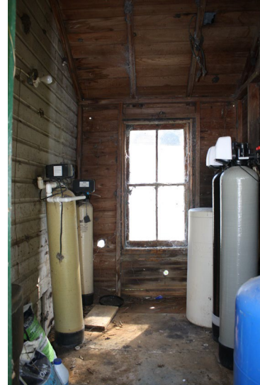
Rear storage room at Double Garage.
