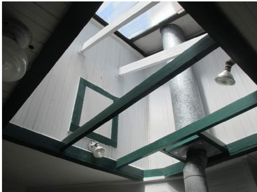
Photograph 3 Skylight within Main House Kitchen
