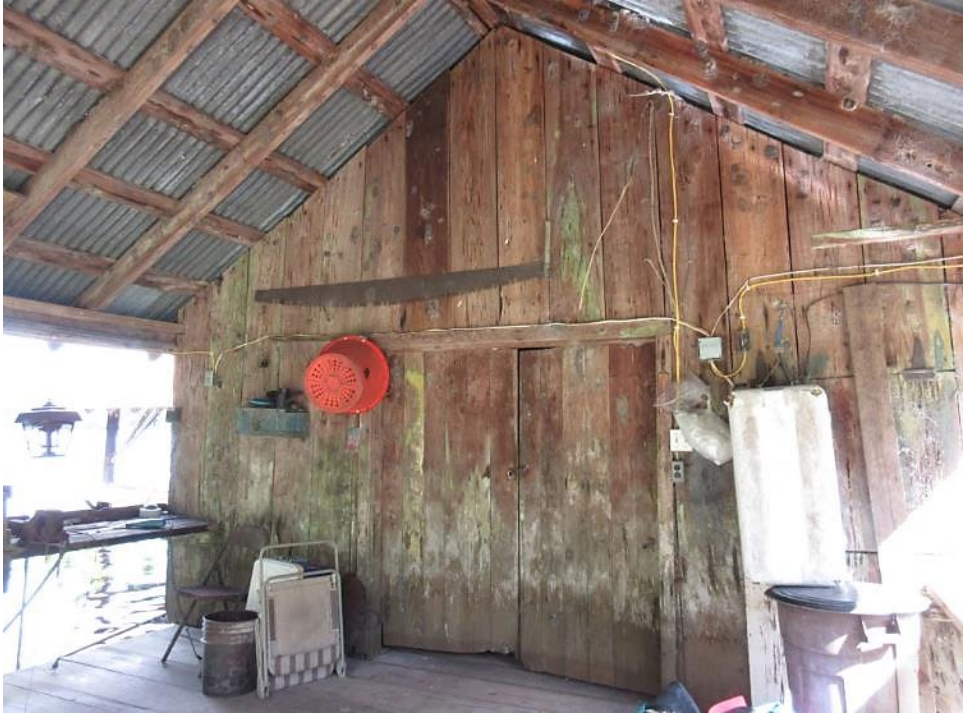
Detail of the front of the storage shed.
