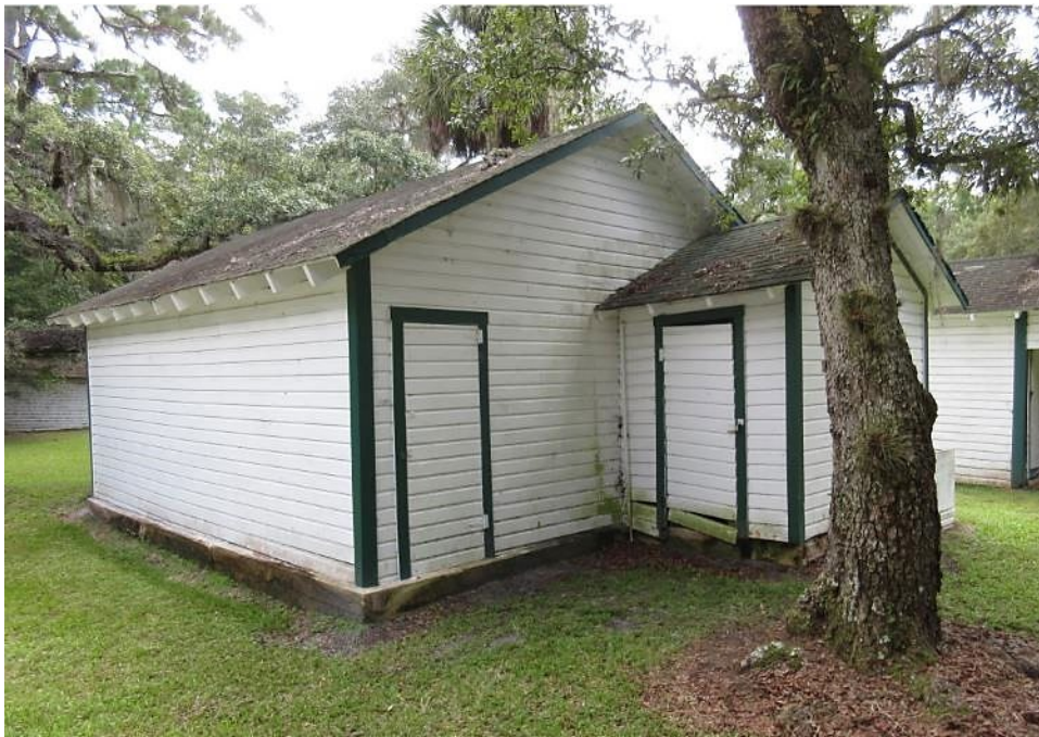
Rear (west) and north facades of the Garage.
