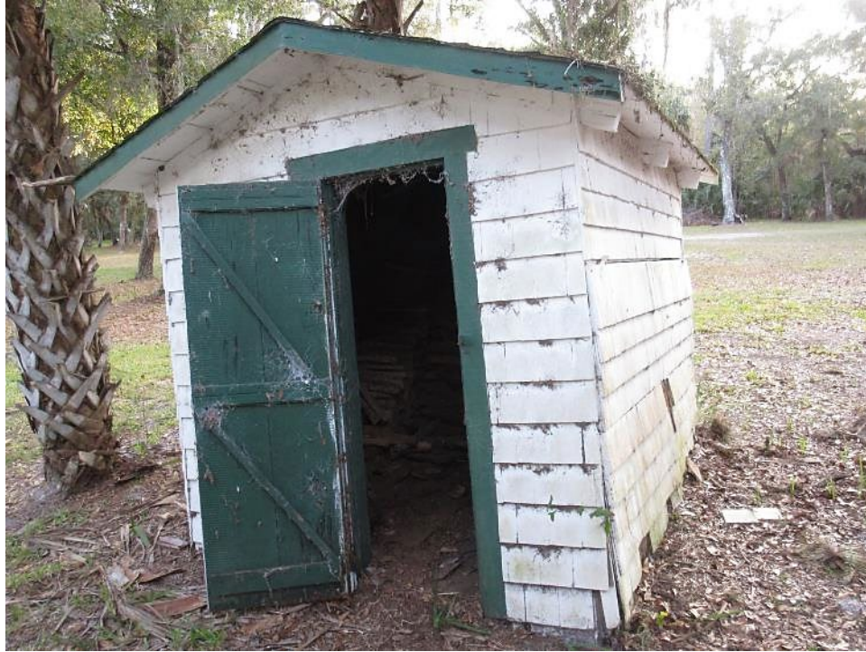
Detail view showing door construction.
