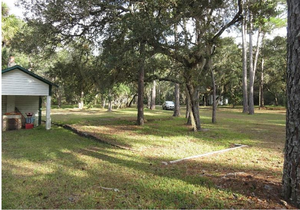
View southeast showing the sloped northwest corner of the Dog Kennel Foundation.
