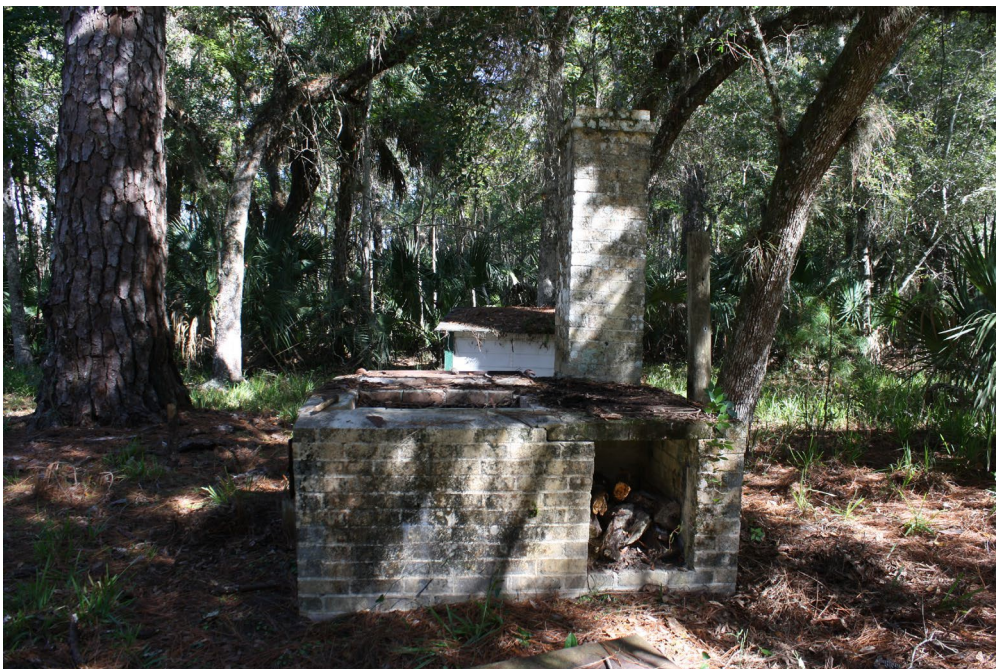
West side elevation of the grill.
