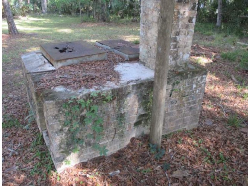
Photograph 2 Biological Growth and Vegetation on Outdoor Grill
