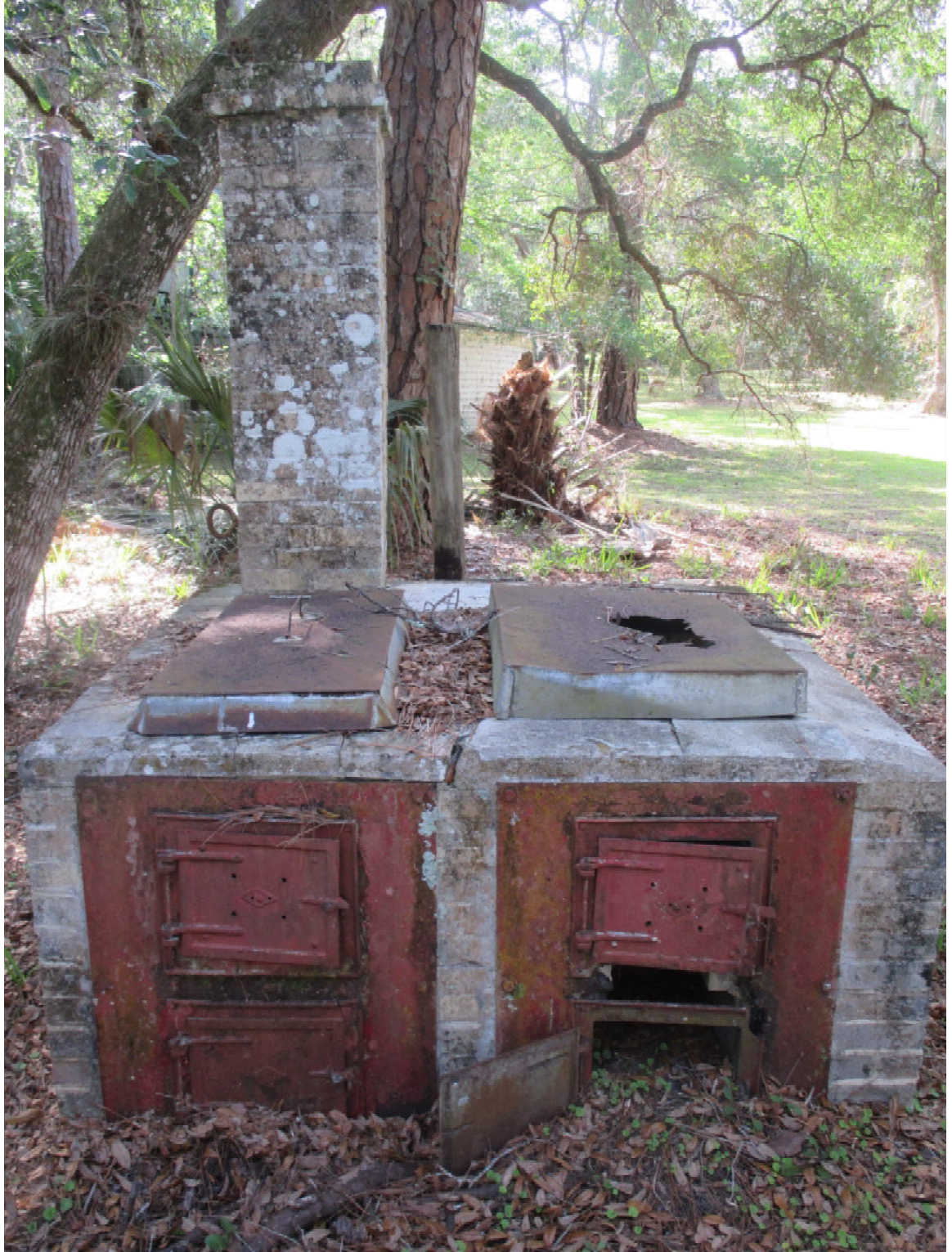
Photograph 1 Overall Outdoor Grill Front
