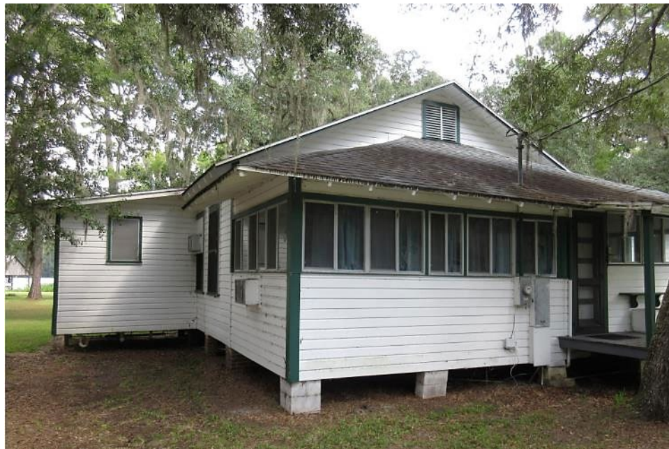
View of the southwest corner of the building.
