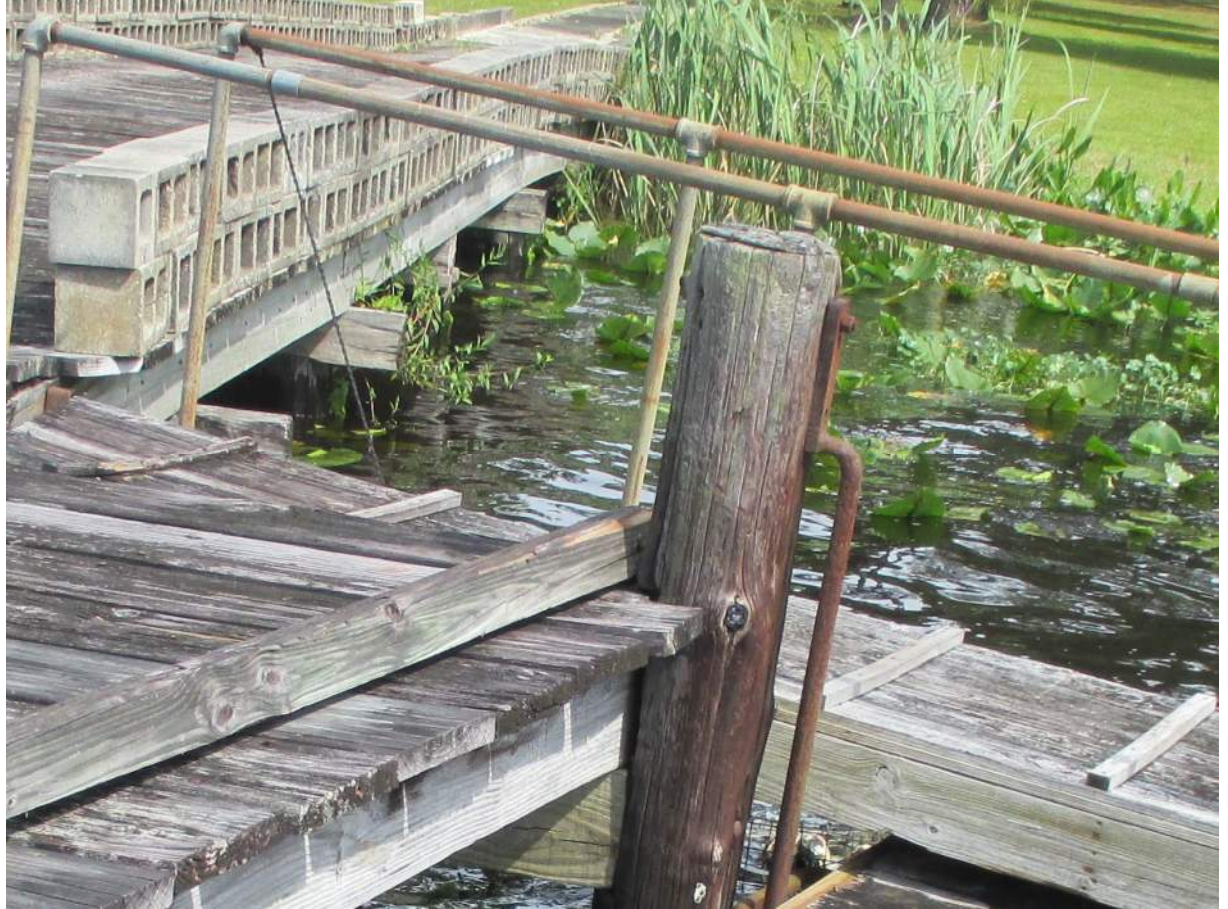
Photograph 11 Perimeter Timber Unattached
