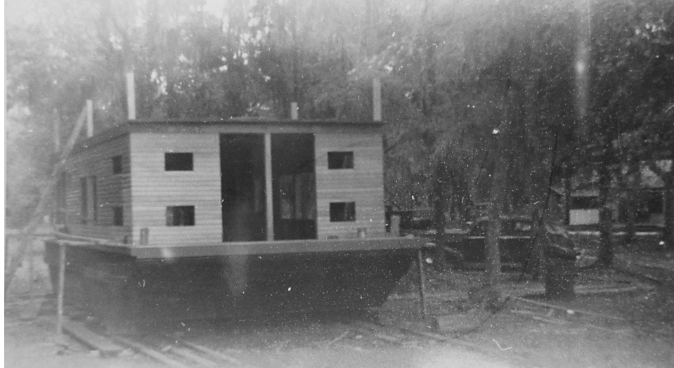
Circa 1939 or early 1940 view of the Houseboat deck under construction. (Photo courtesy Bob McKinstry)
