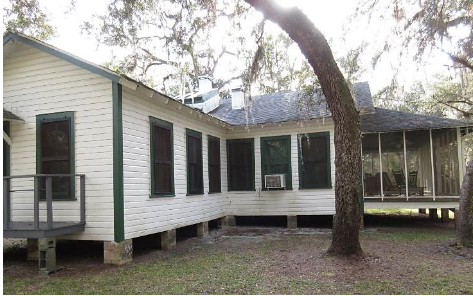
View of the northeast portion of the building with the dining room addition at left.
