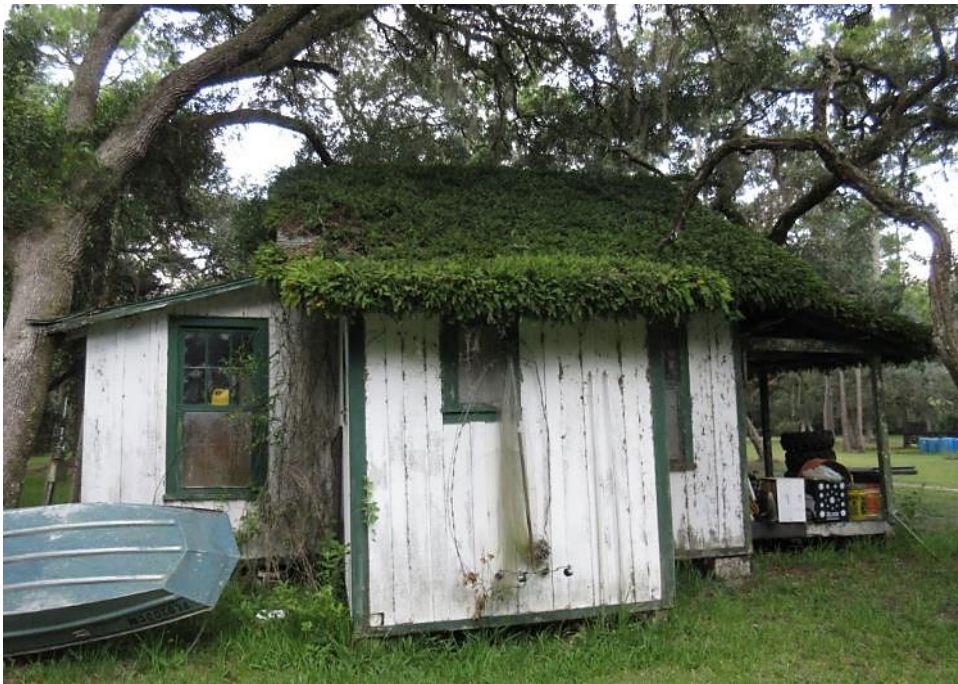
East façade of the Cook's House.
