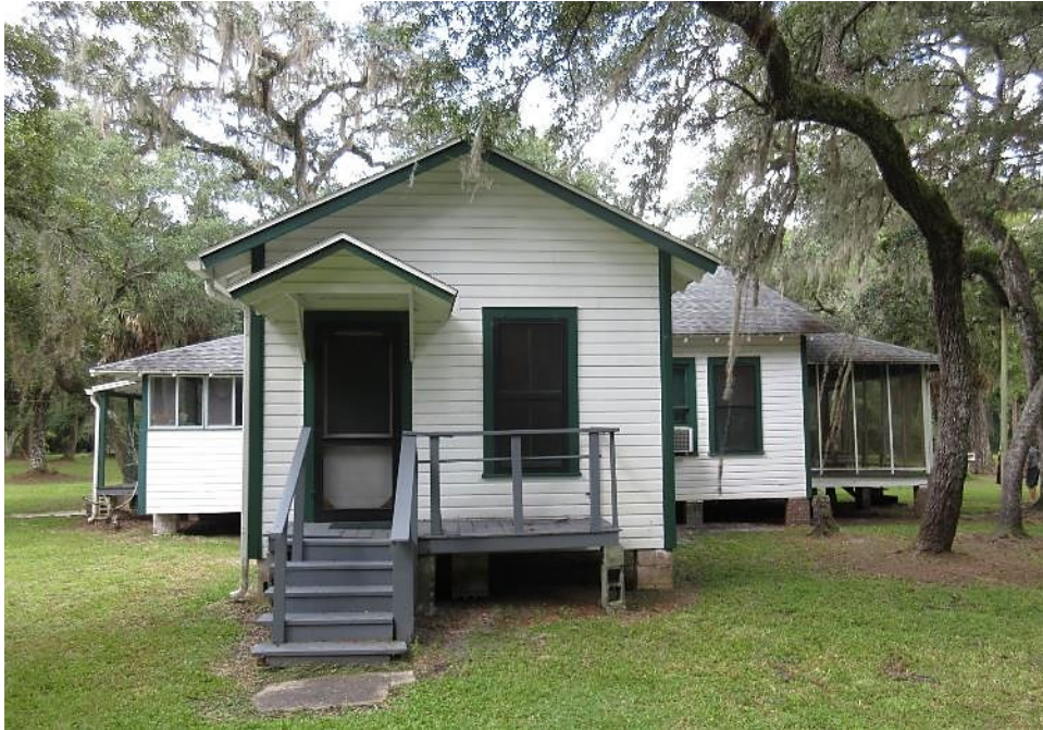
View of the east entry to the dining room.
