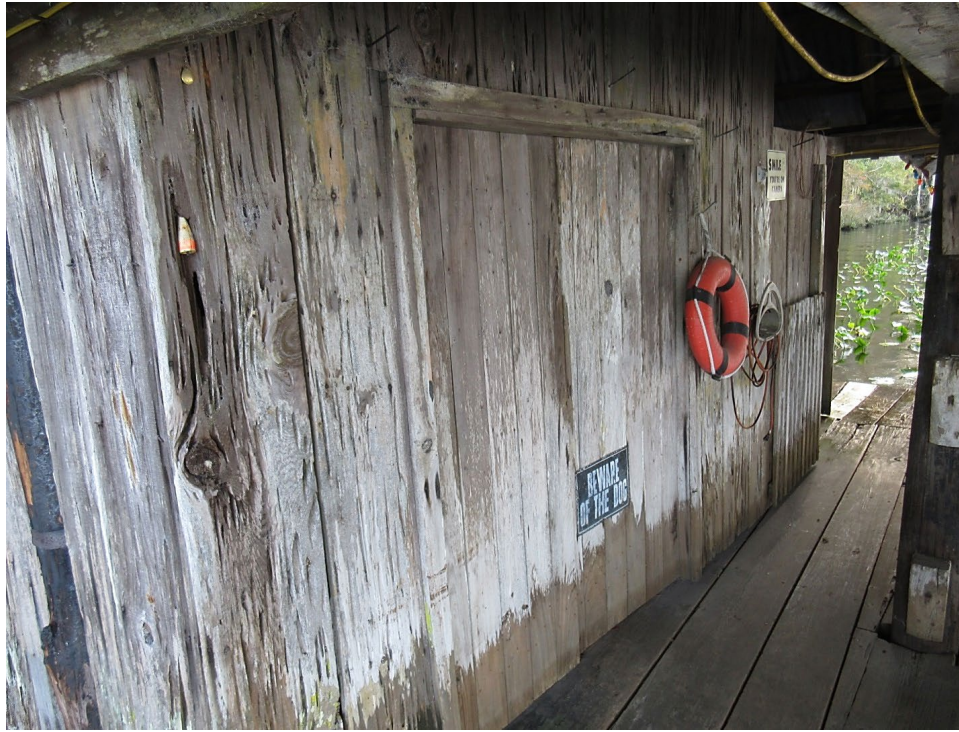
View west along the walkway at the rear of the Boathouse.
