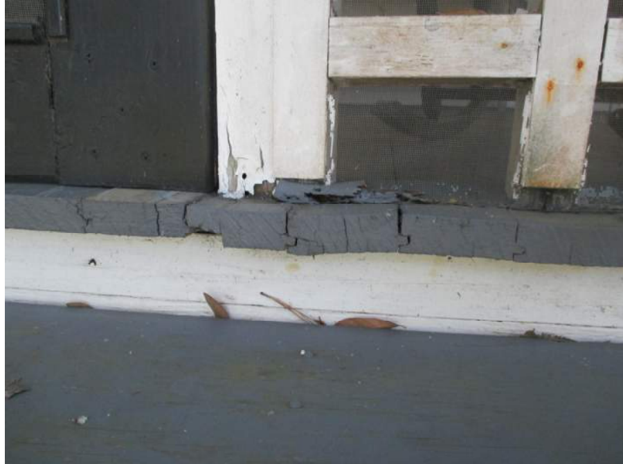
Photograph 14 Water Damaged Decking at Main Entry Porch
