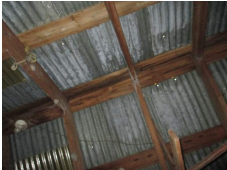
Photograph 4 Underside of Metal Roofing
